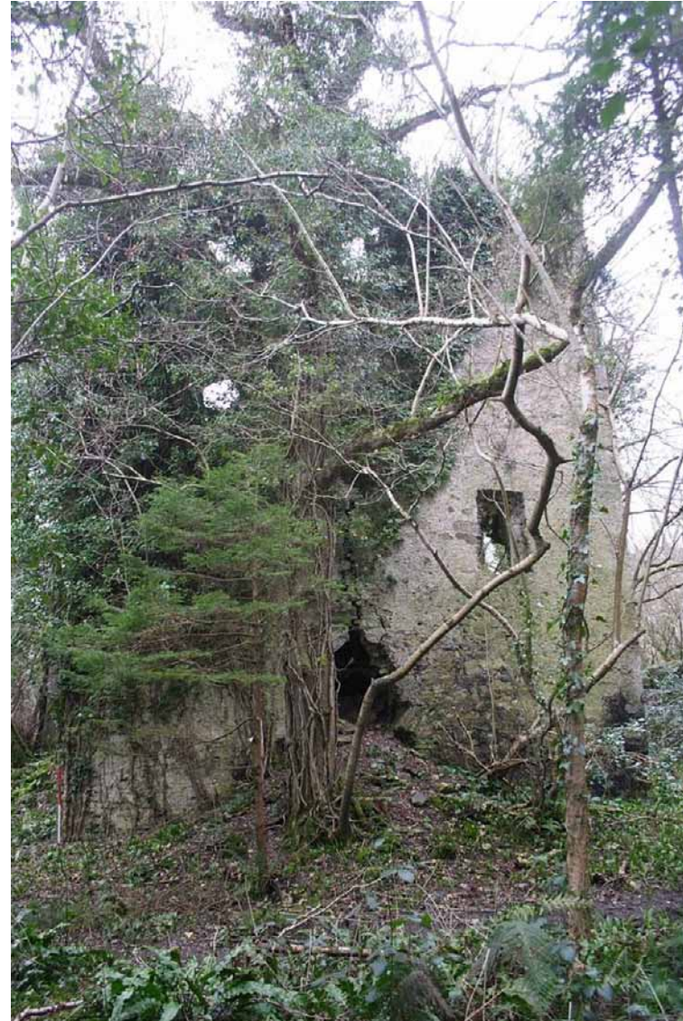
Photo 8: The eastern face of the Eastern Tower. 1m scale.
