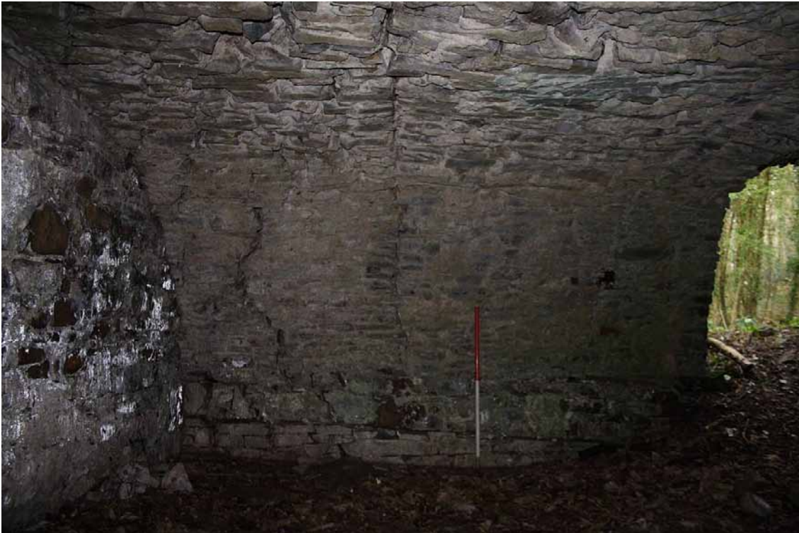
Photo 33: Join in the ceiling of the undercroft. View looking north. 1m scale.
