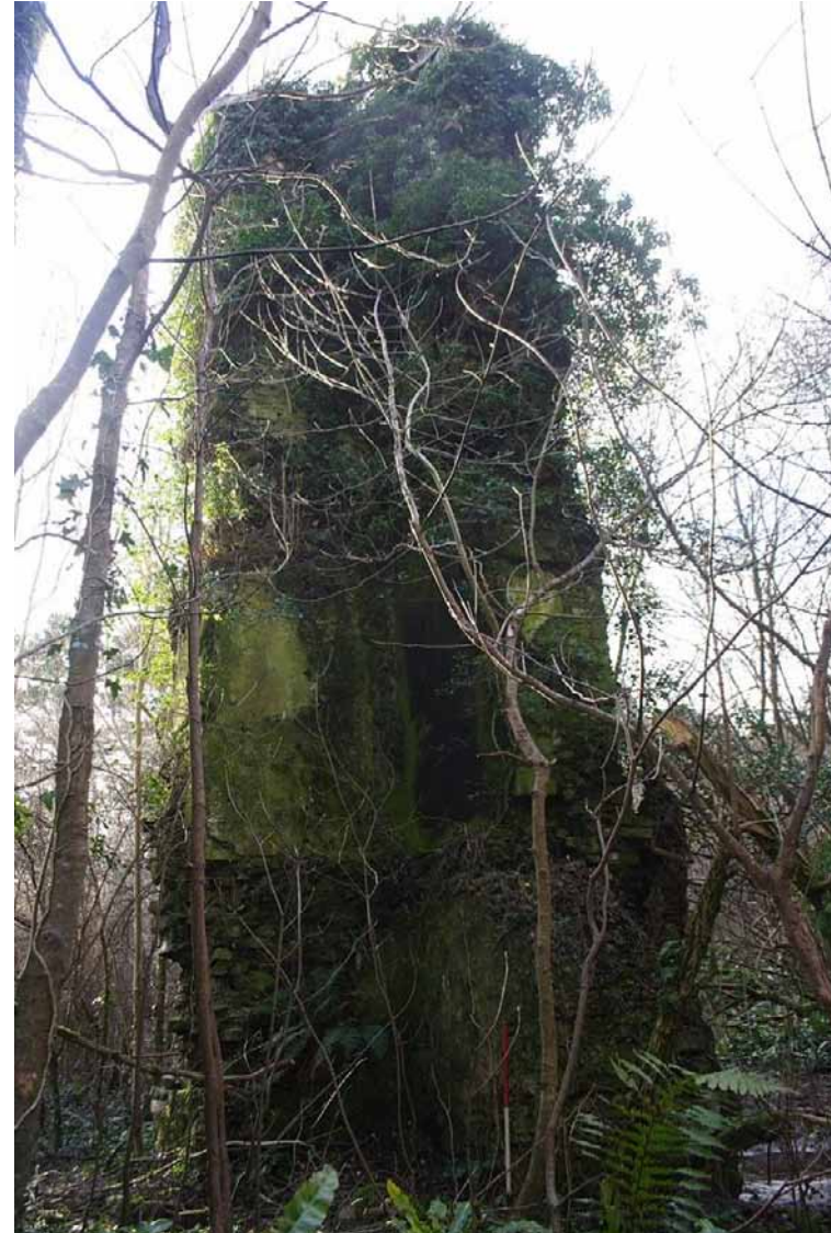
Photo 20: Interior of the northern part of the Western Tower, also showing the rendered side of a window in the western wall at 1 st floor level. 1m scale.
