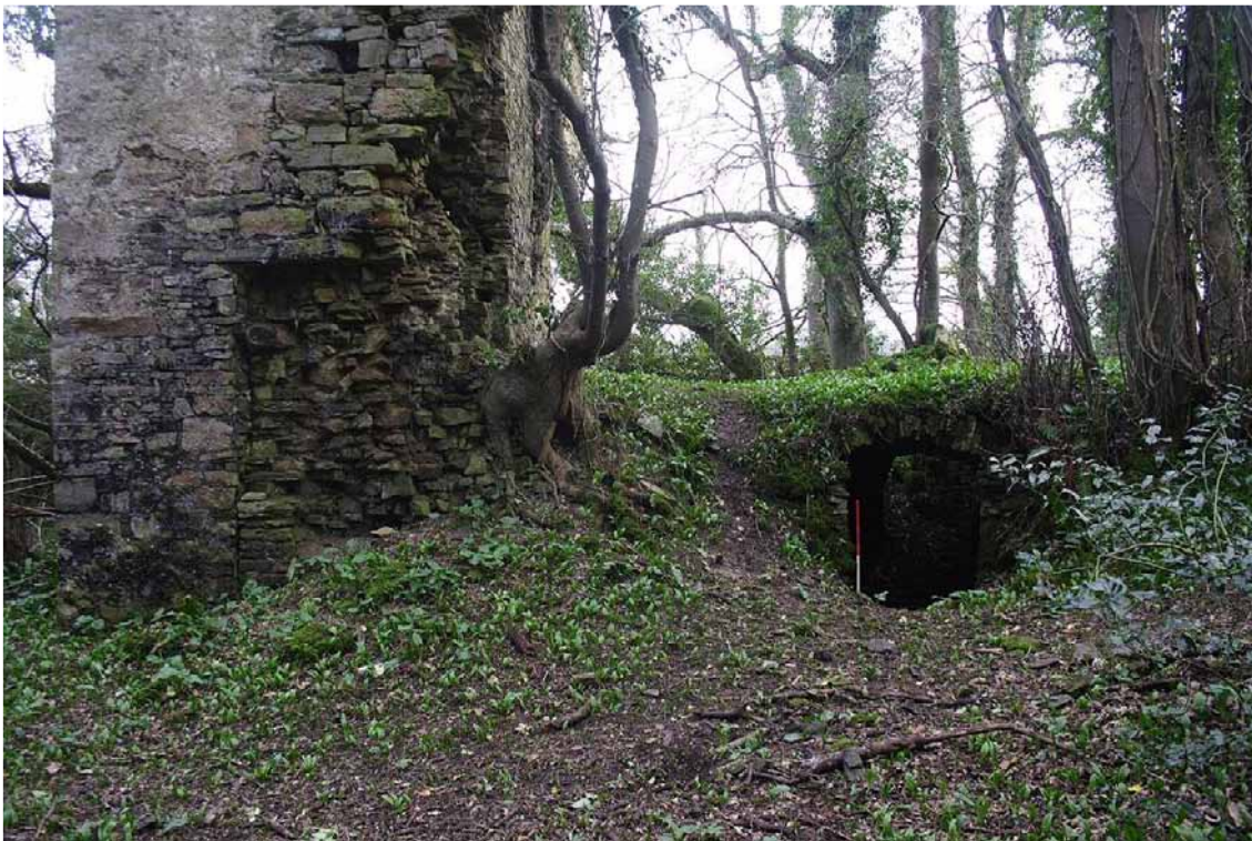
Photo 26: View south towards the Eastern Tower and main entrance into the undercroft. 1m scale.
