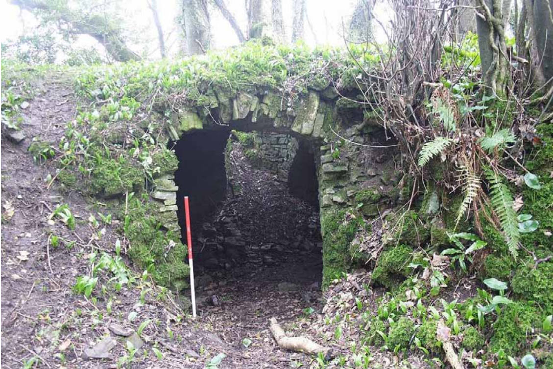
Photo 27: Main entrance to the undercroft from the north. 1m scale.
