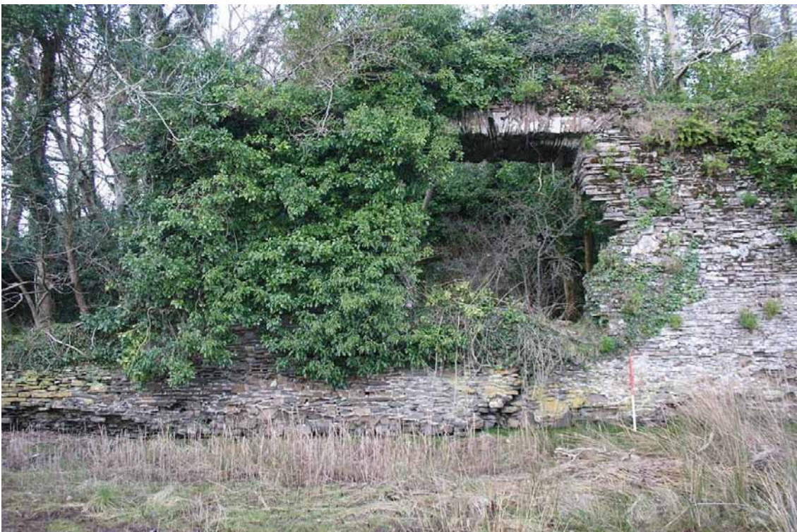
Photo 38: Main entrance into the Garden Enclosure viewed from the rivers edge. 1m scale.
