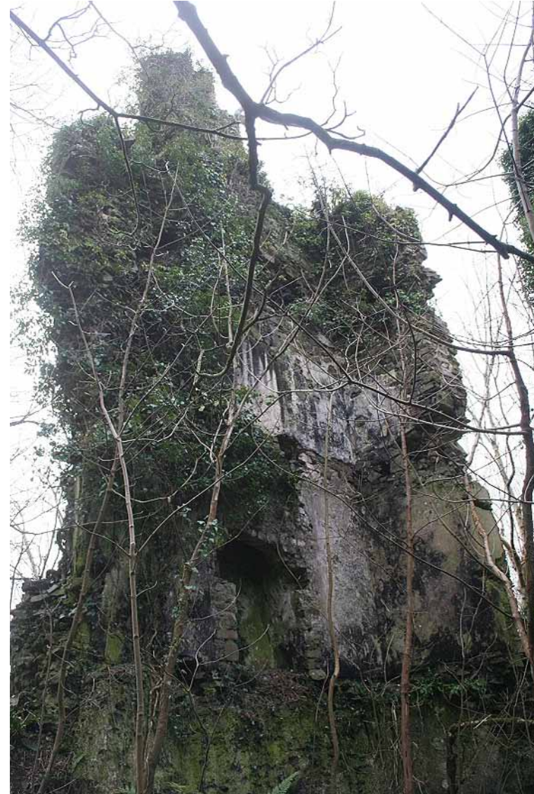
Photo 18: Interior of the southern section of the Western Tower. 1 st floor fireplace visible, with remnants of chimney stacks at the top.
