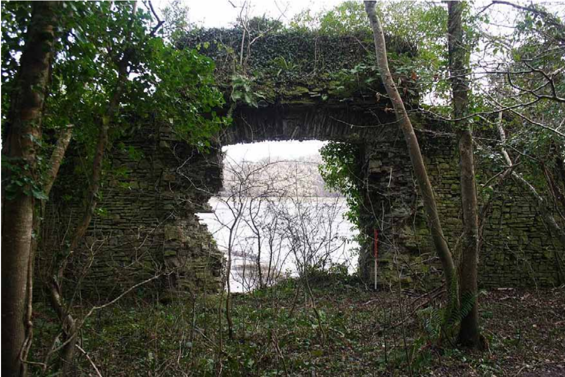
Photo 37: Main entrance through the southern wall of the Garden Enclosure, viewed from the north. 1m scale.
