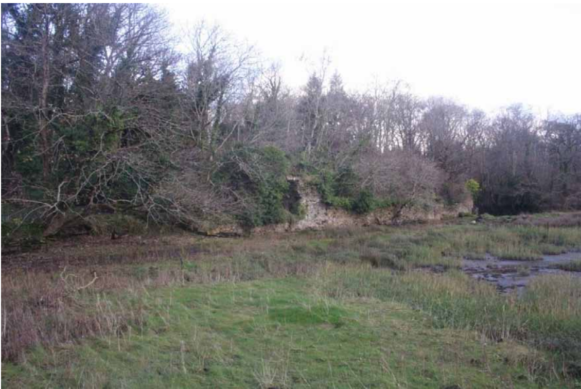
Photo 34: Looking northeast at the southern wall of the Garden Enclosure.
