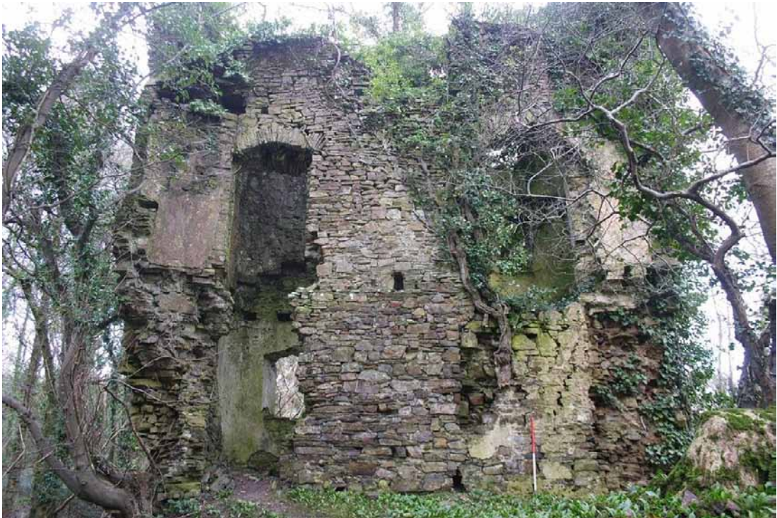
Photo 6: The western face of the Eastern Tower. 1m scale.
