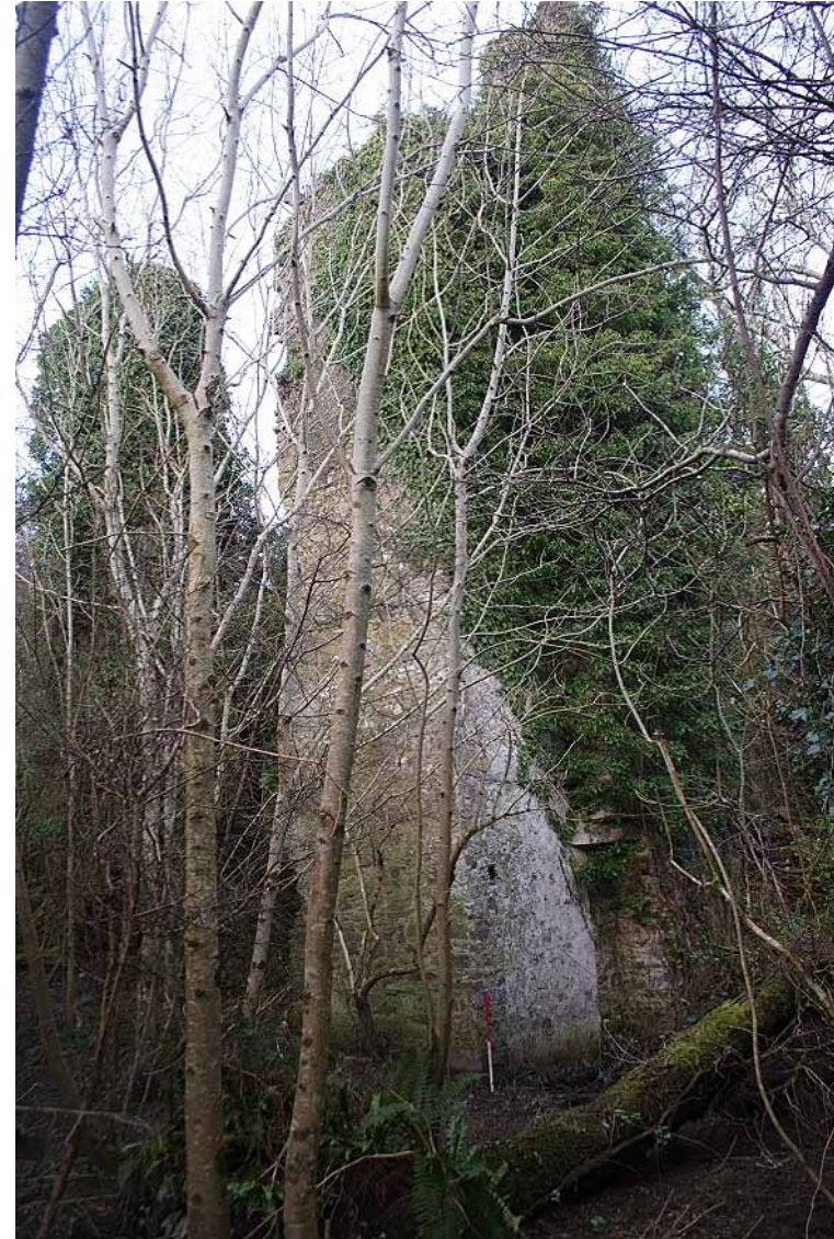
Photo 14: General view of Western Tower, looking northeast. 1m scale.
