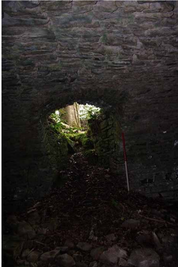
Photo 31: Opening/entrance in southern wall of the undercroft
