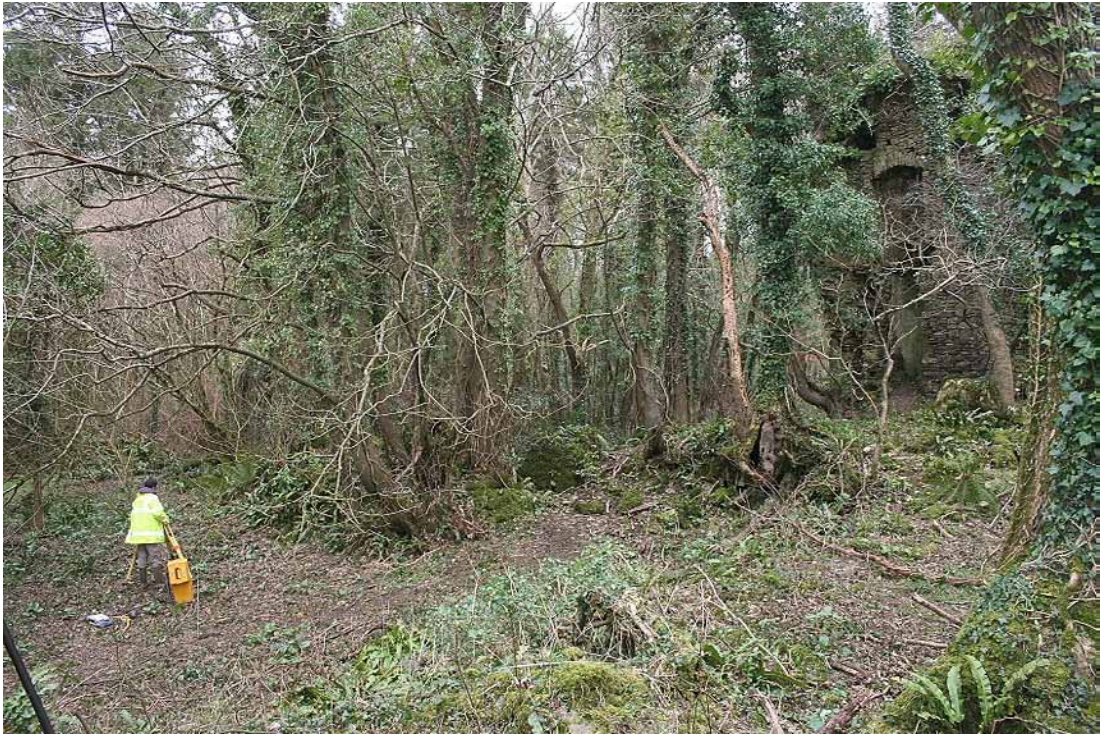
Photo 3: General view of the main hall area. The east tower is visible on the right.
