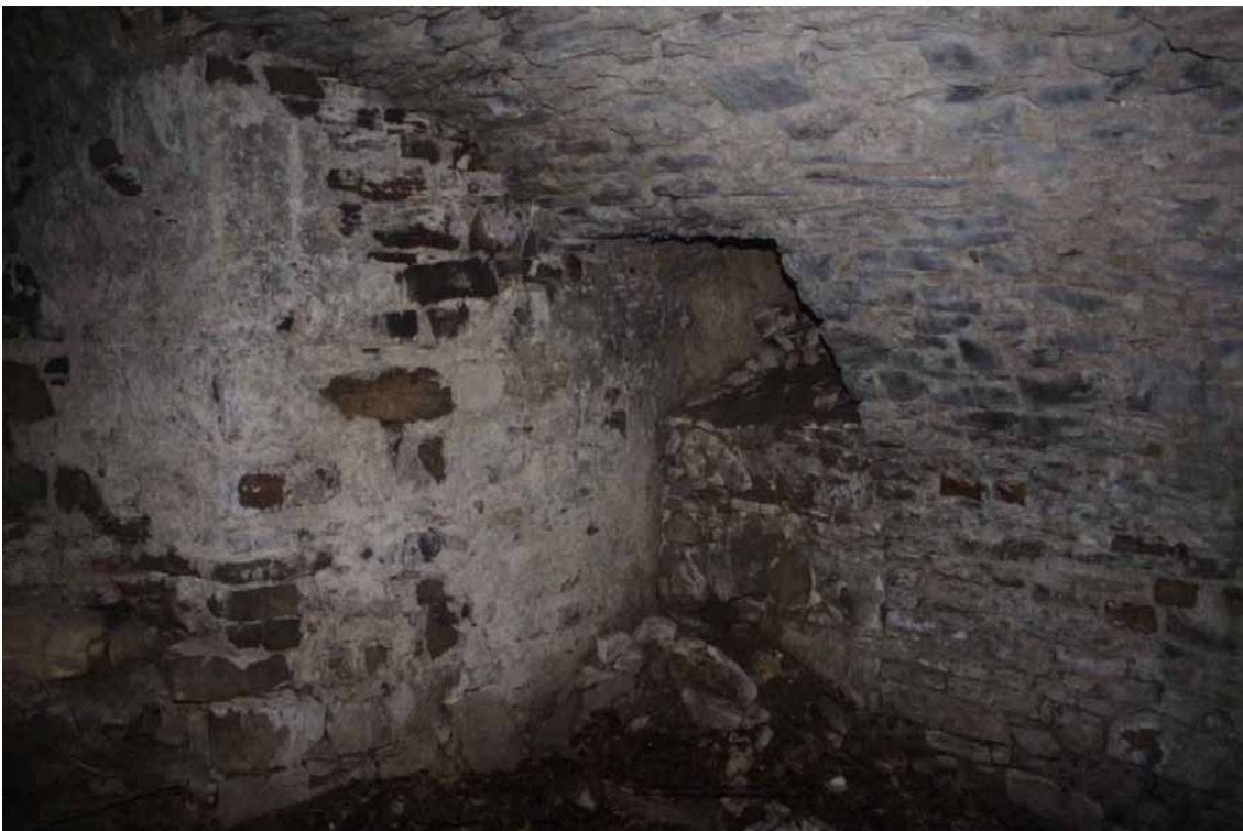
Photo 30: Blocked opening in the southeast corner of the undercroft.
