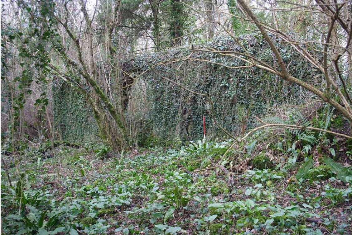
Photo 49: Eastern wall of the Northwest Enclosure, looking northeast. 1m scale.
