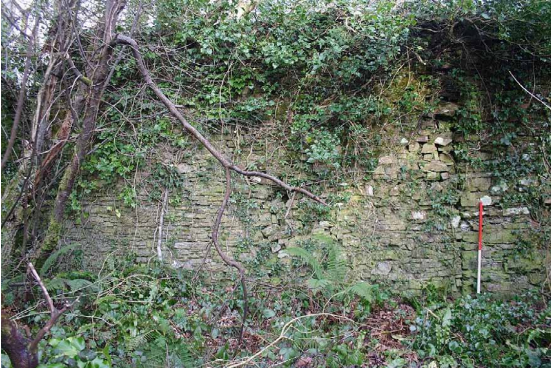
Photo 41: Interior of the eastern wall of the Garden Enclosure, showing the vertical joint of a possible entranceway. 1m scale.
