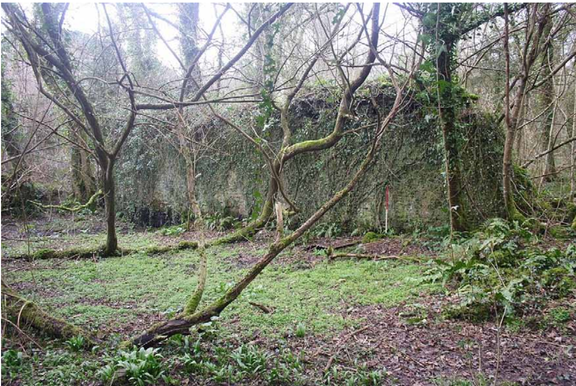
Photo 50: Northern wall of the Northwest Enclosure, looking northwest. 1m scale.
