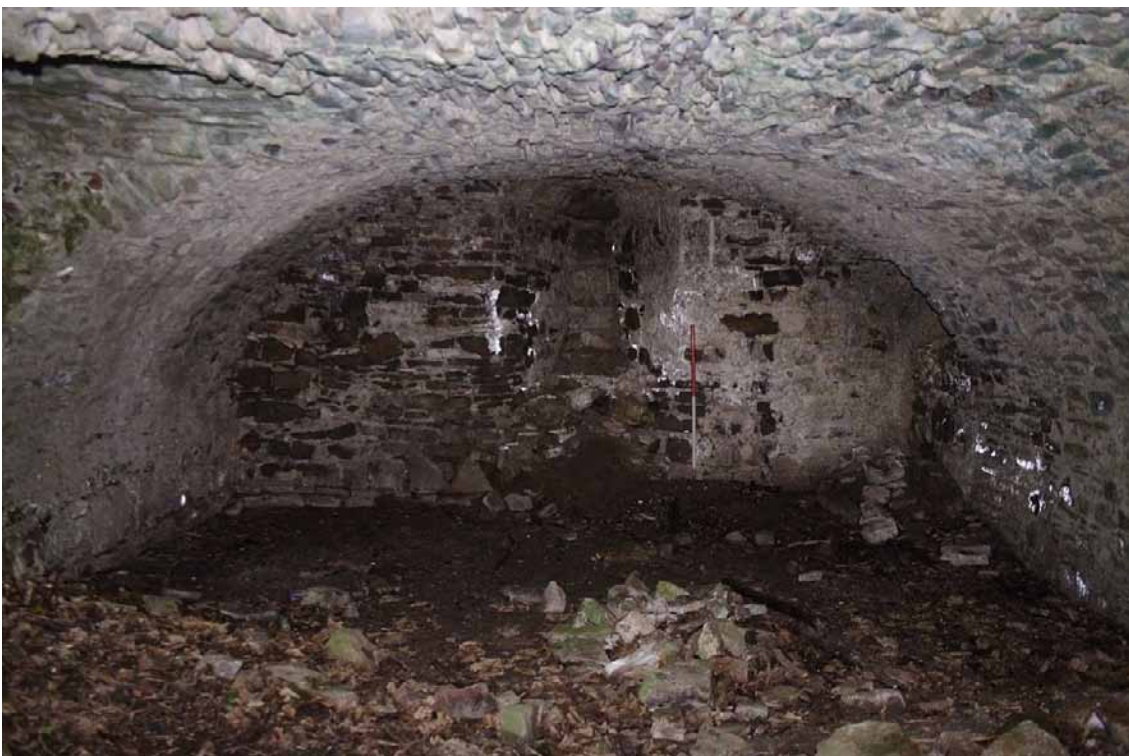
Photo 28: Interior of the undercroft, looking east. 1m scale.
