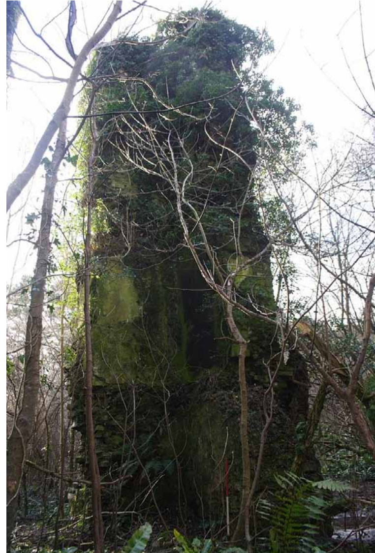
Photo 20: Interior of the northern part of the Western Tower, also showing the rendered side of a window in the western wall at 1 st floor level. 1m scale.
