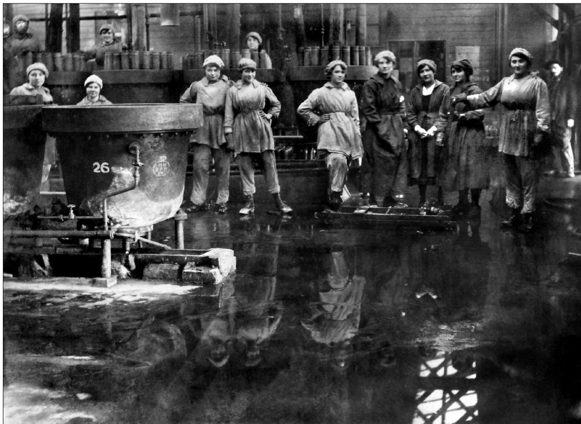
Figure 21. Melting HE (high explosive) out of shells. (National Archives, MUN 5-155)
