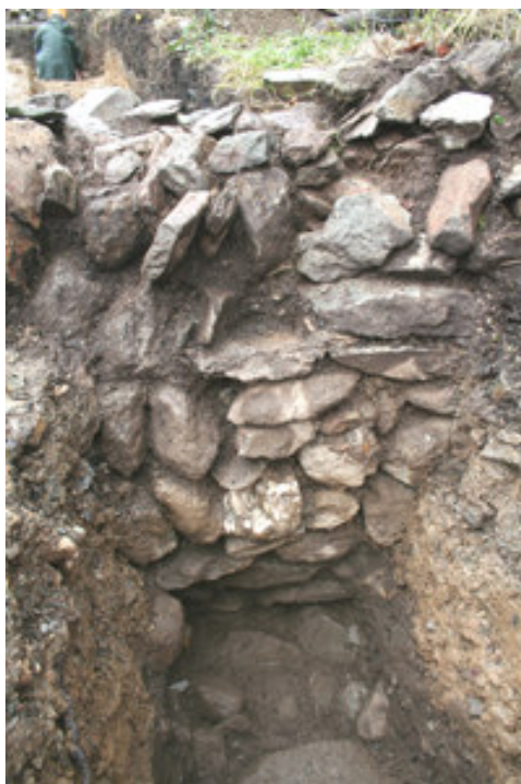
Photo 17: Trench 2, looking southwest, showing north face of the castle/pound wall.
