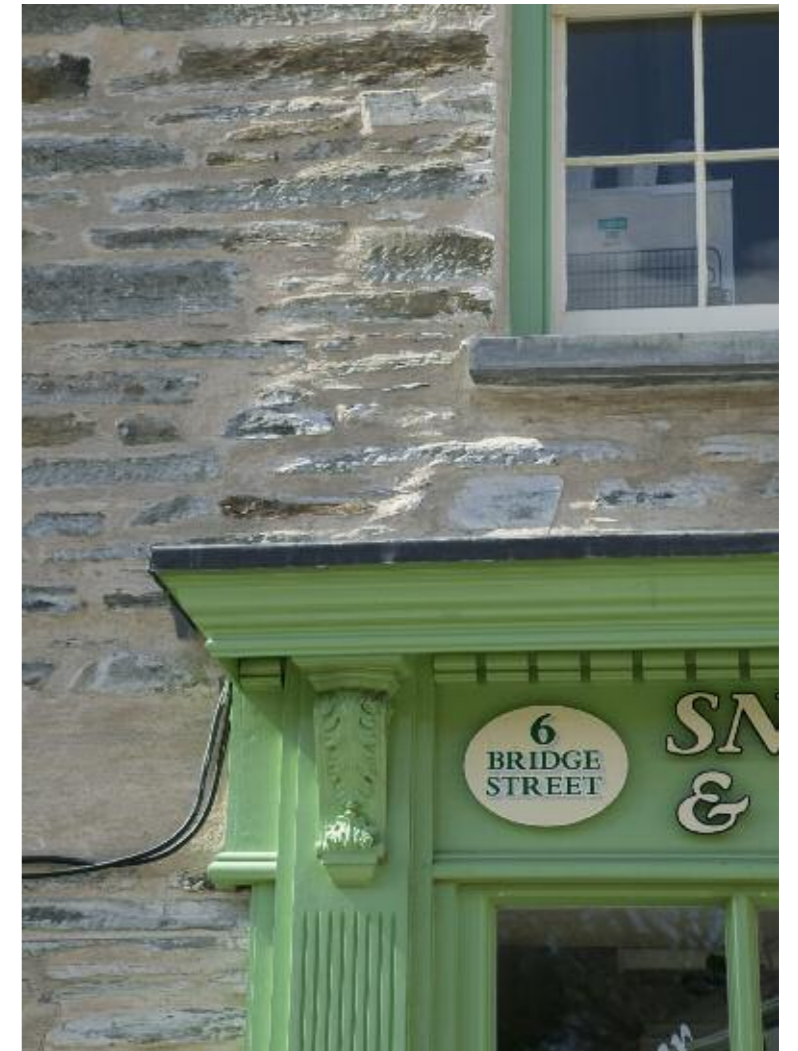
The extensive use of the distinctive grey Teifi slate can be seen throughout Cardigan, in prominent buildings, such as the Shire Hall (left), Guildhall (above) and Glenroy House on Bridge Street (right).
