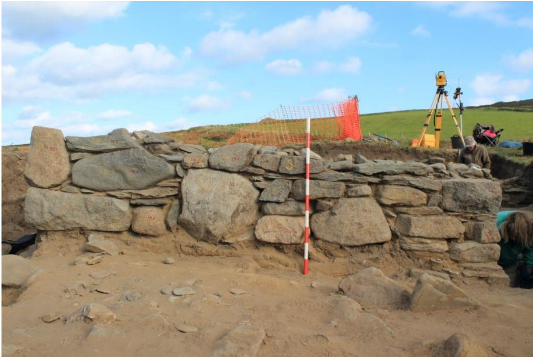
Photograph 5. The external rebuilt façade of the south wall of the chapel (511). Scale 1m
