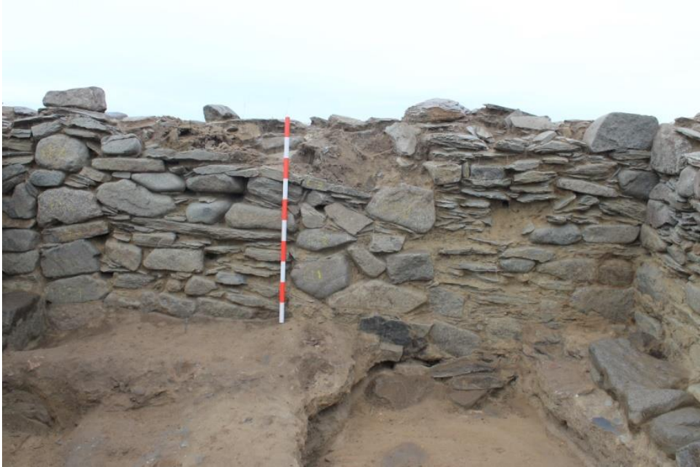
Photograph 3. The internal west wall of the stone-built chapel showing the blocked doorway 83/176, the wall to the north of the doorway (82/177) and the wall to the south (174/175). Scale 1m
