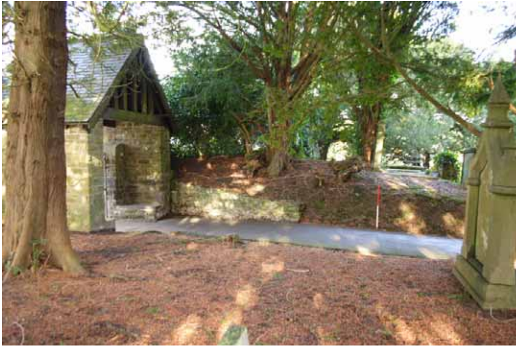
View of defensive bank by church yard entrance.
