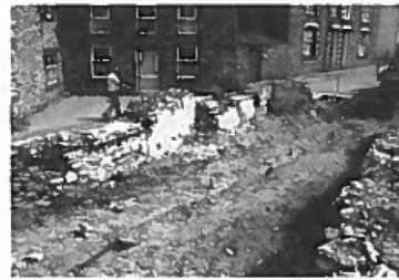
16. Foundation trench for new boundary wall
