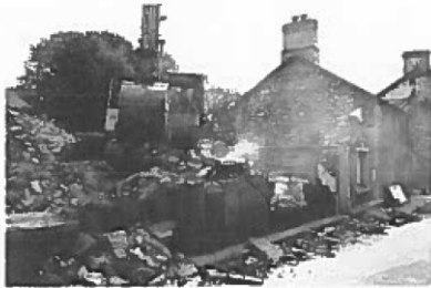
15. Gelli-gron during final phases of demolition
