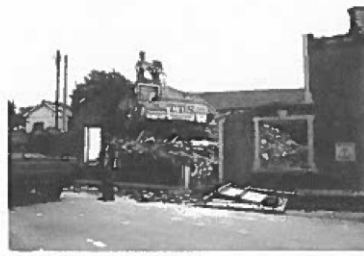
14. Gelli-gron during final phases of demolition work
