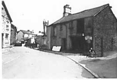
13. Gelli-gron during final phase of demolition
