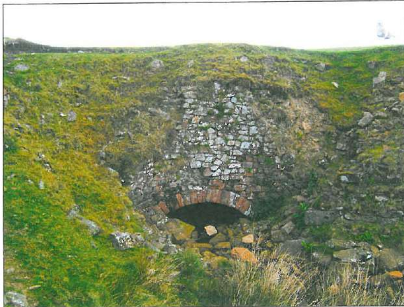
Plate 11: Single Arched Bridge IWT007/012 on Causeway IWT007/024
