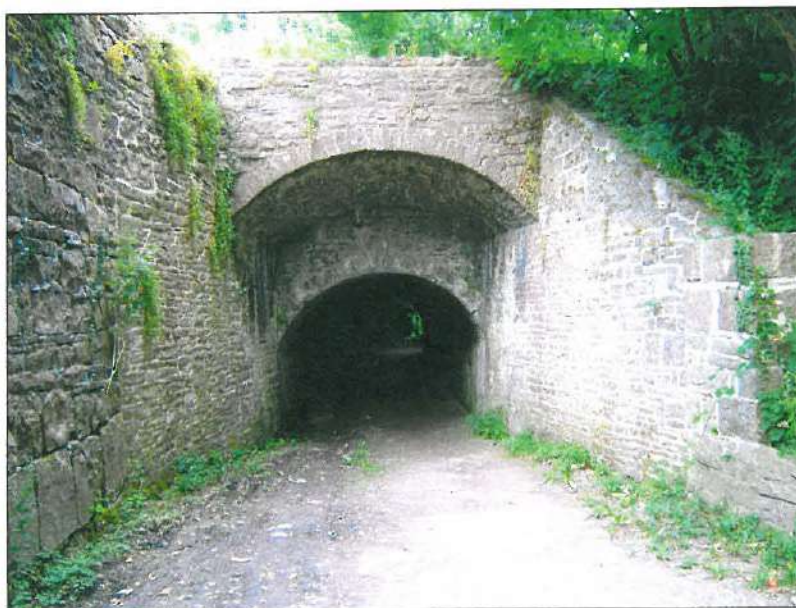
Plate 5: Gilwern Embankment (SAM MM251)
