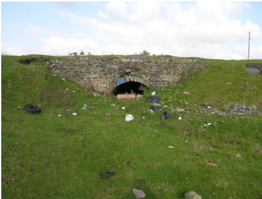
Plate 57. Culvert EA066.08 carrying the B4256 across area of workings between EA066.03 and EA066.02, view to north
