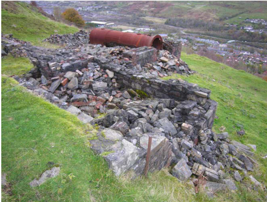
Plate 60. Remains of northern Engine House EA071.07 with boiler in situ , view to west
