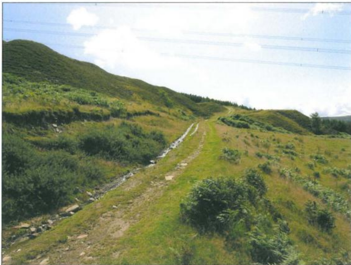
Plate 15. Tramroad NPRN 262599 approaching Quarry NPRN 262598, view to south-south-east
