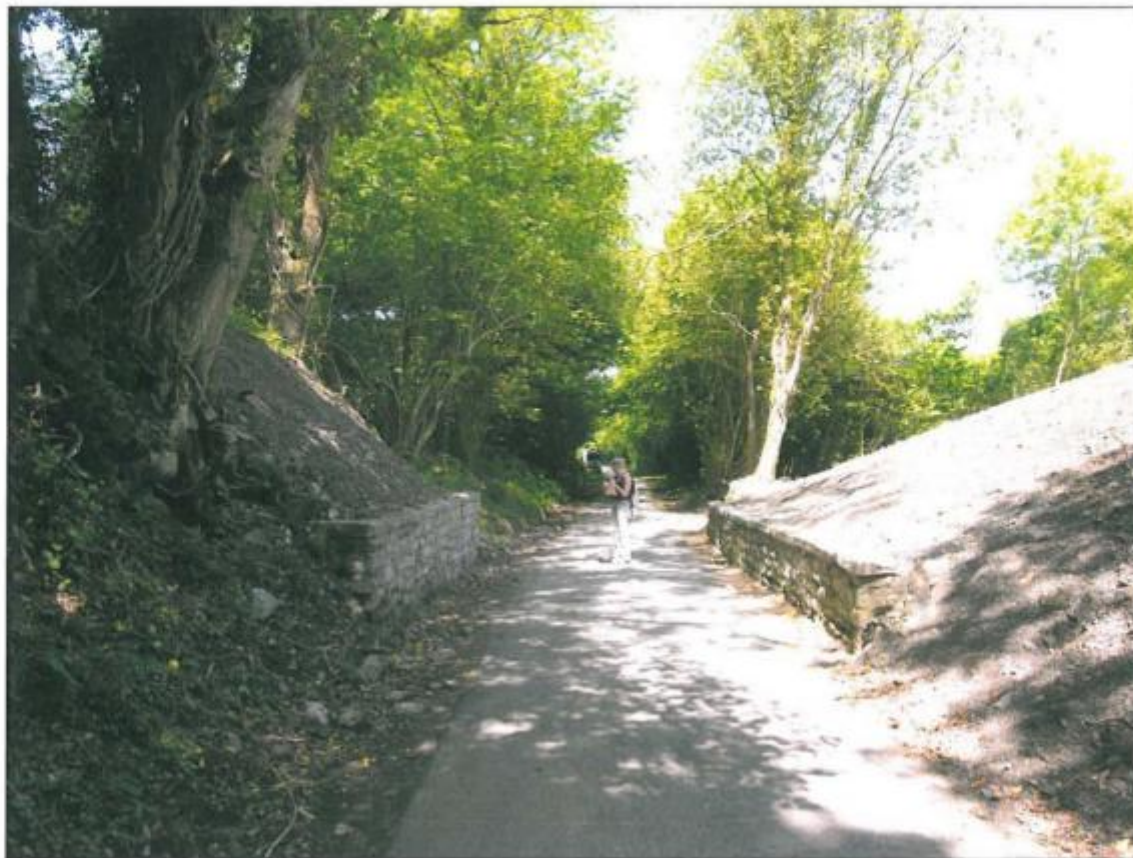
Plate 18. Gamlyn tramroad and abutments EA004.02, view to the north
