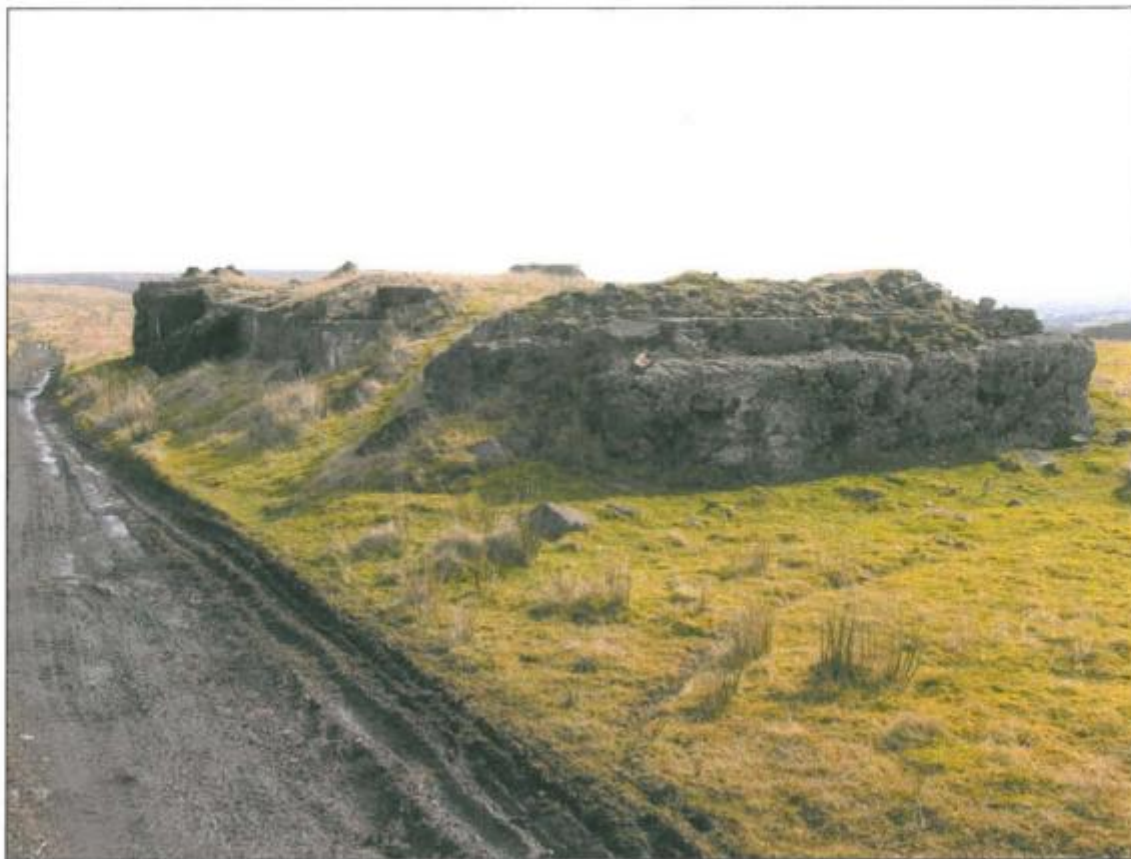
Plate 70. Concrete Structure EA082.10 (coke ovens shown on 1st edition), view to the east
