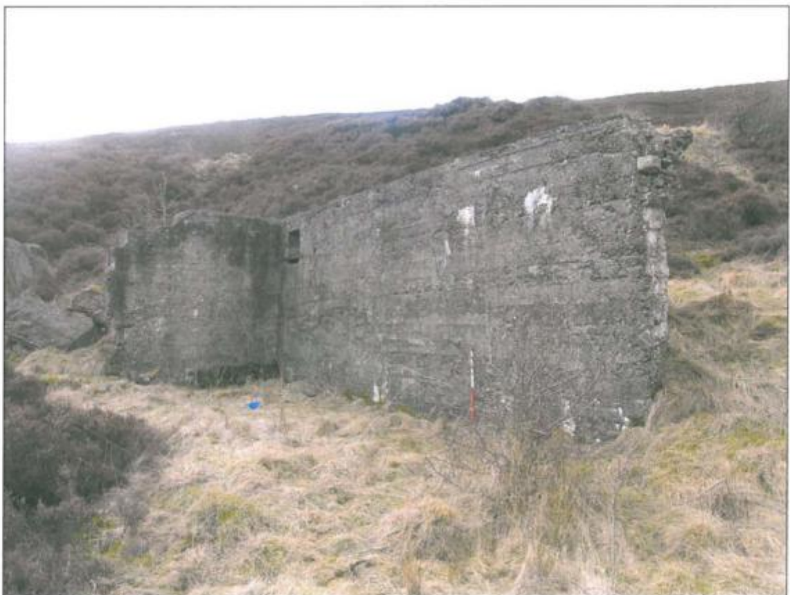
Plate 86. Concrete structure EA093.126, view to south-west
