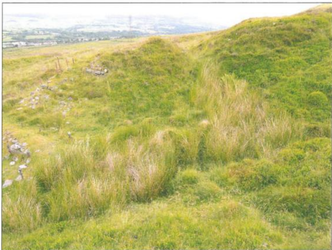
Plate 23. Approach to collapsed Drift mine entrance EA005.08 and eastern machinery mount, Craig Colliery, EA005.09, view to the east
