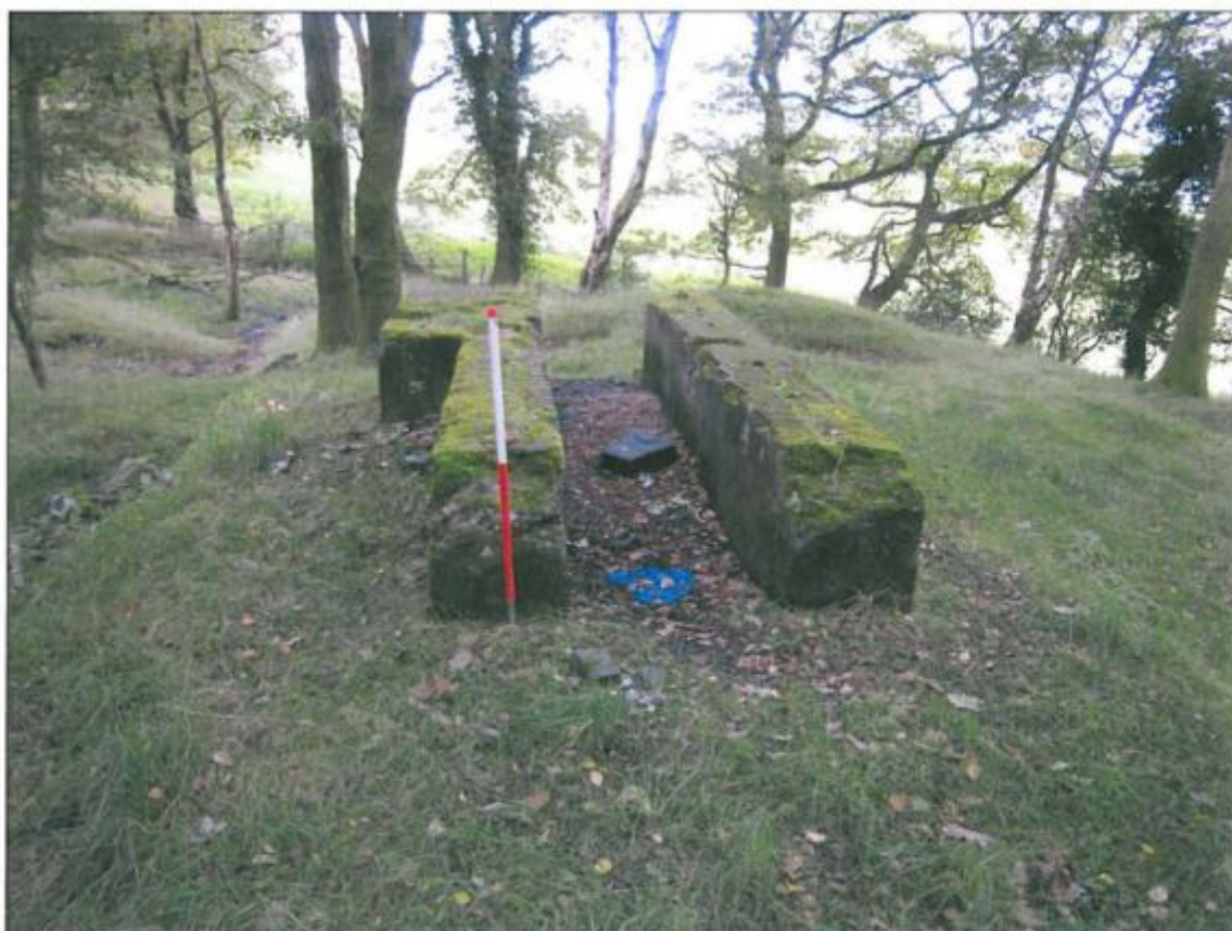
Plate 33. Concrete structure EA010.22, view to the west
