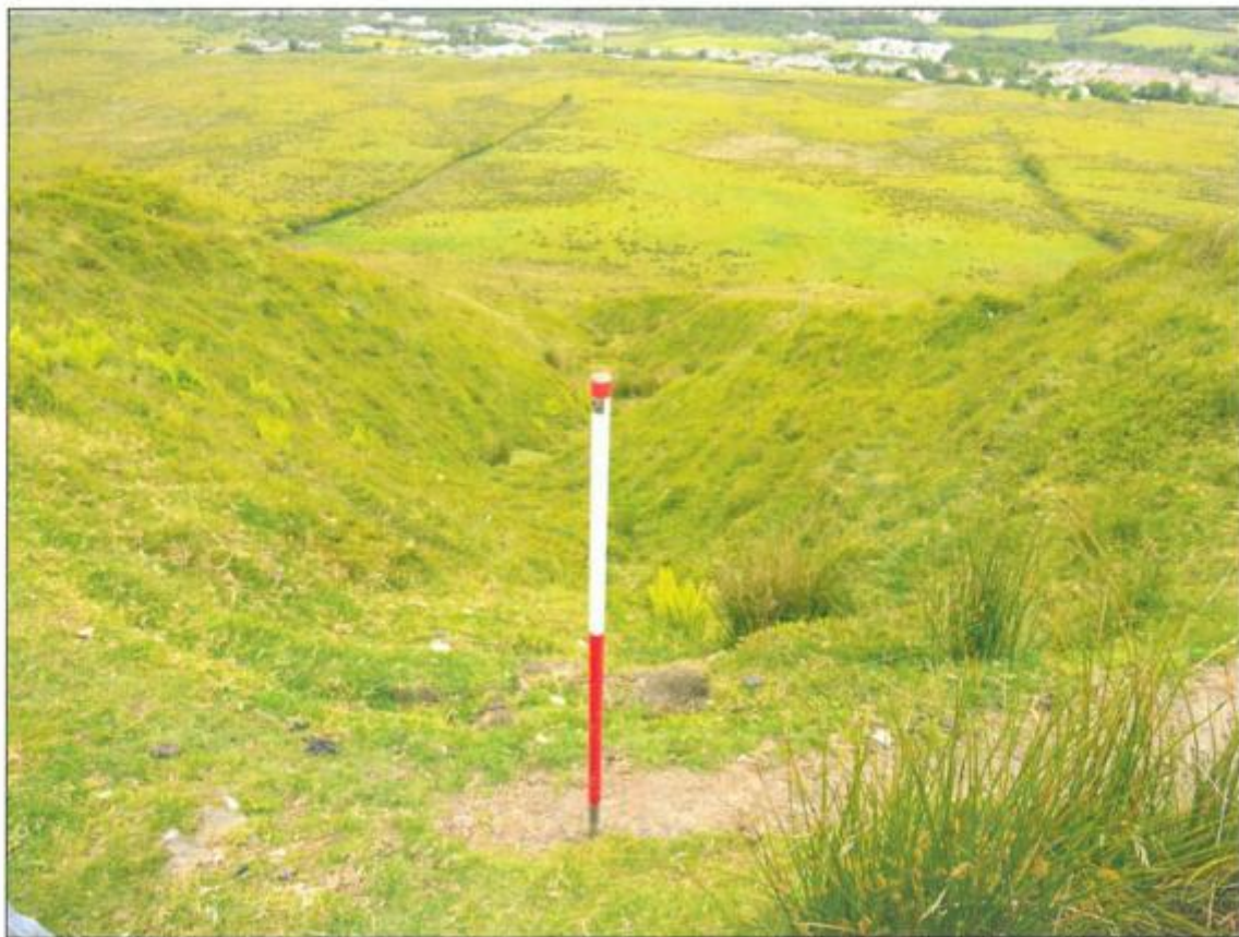
Plate 22. Major scour or gully, EA005, view to the north
