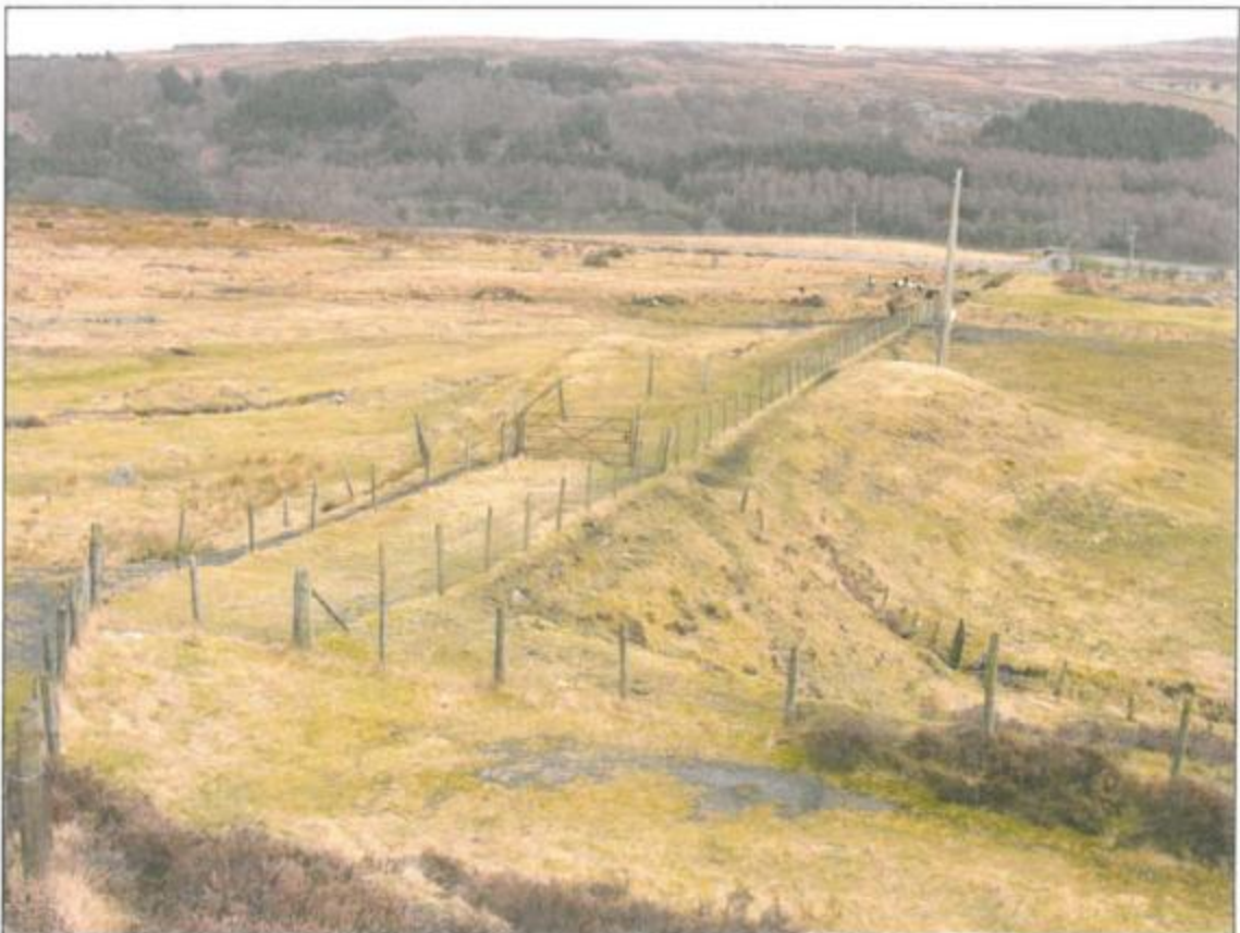
Plate 90. Varteg Incline EA093.124, middle surviving section, view to east
