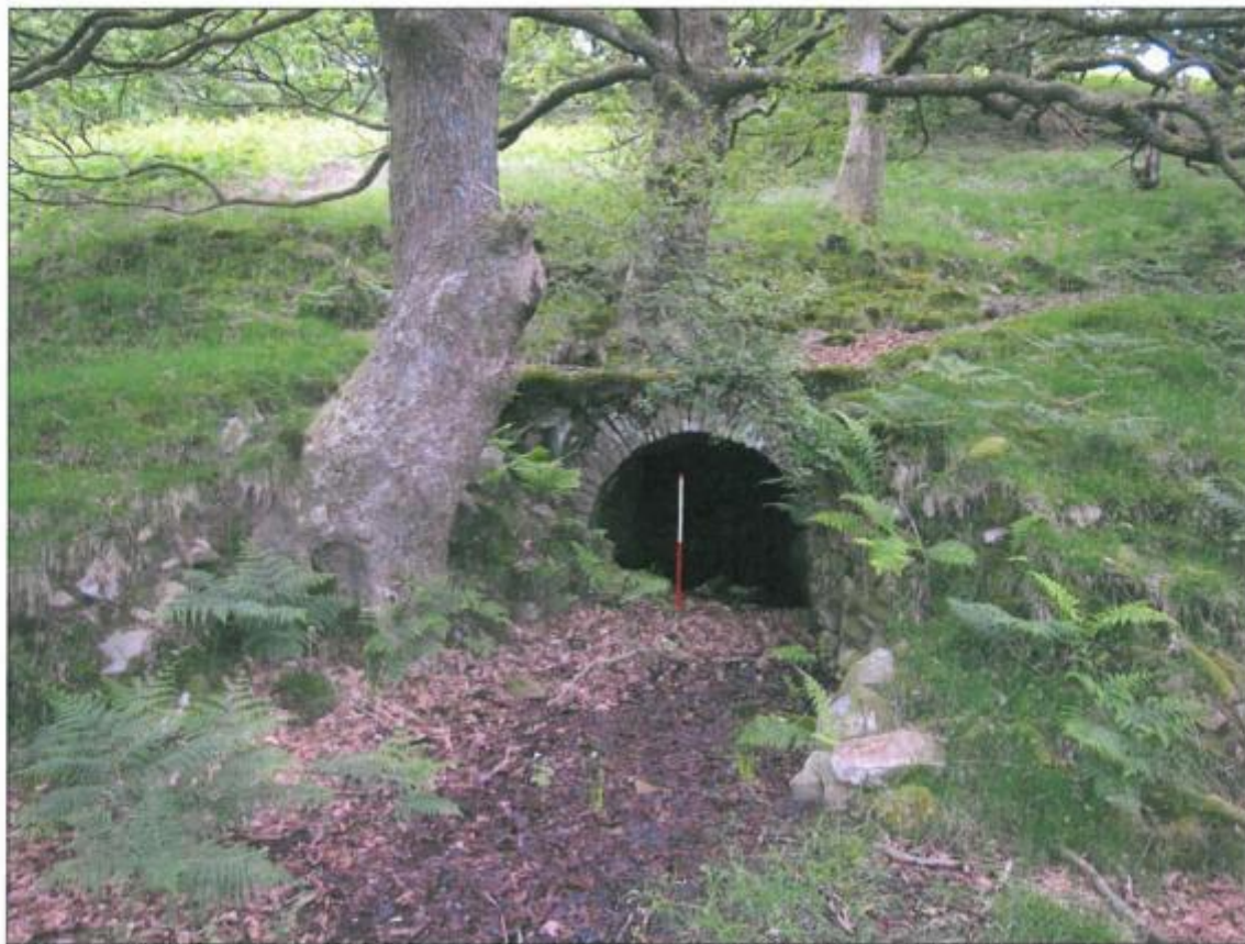
Plate 39. Level entrance EA026.01, view to the north
