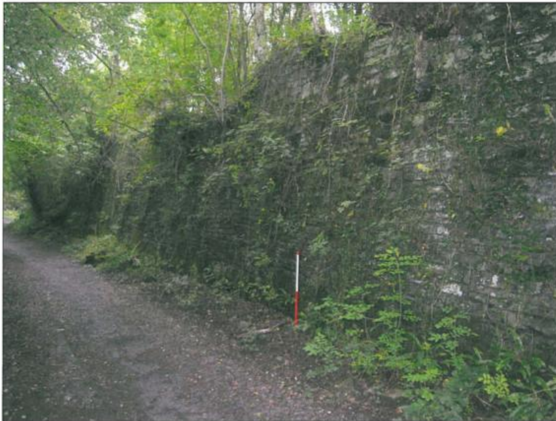
Plate 25. Masonry revetment, Tunnel Pit tramroad, EA006, view to the north-west
