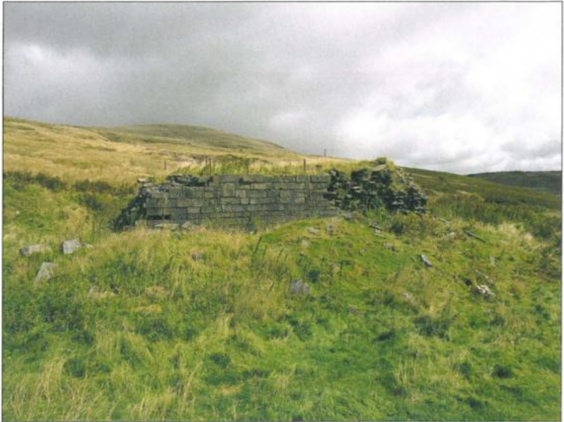
Plate 12. Engine House EA001.69, view to the north-west
