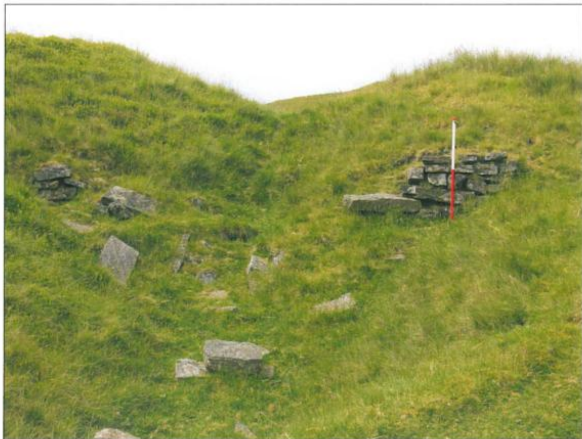
Plate 9. Bridge abutment over tramroad NPRN 262419, view to the north
