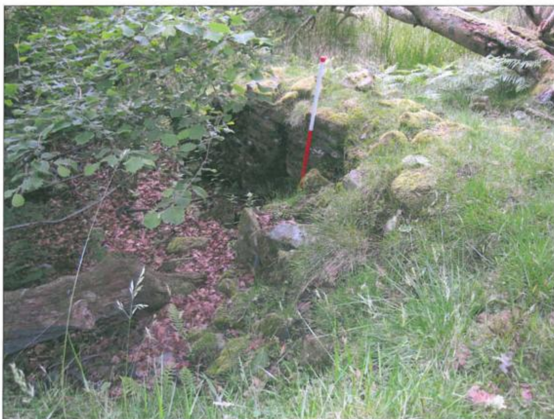
Plate 40. Interior of shaft structure EA026.13, view to the west
