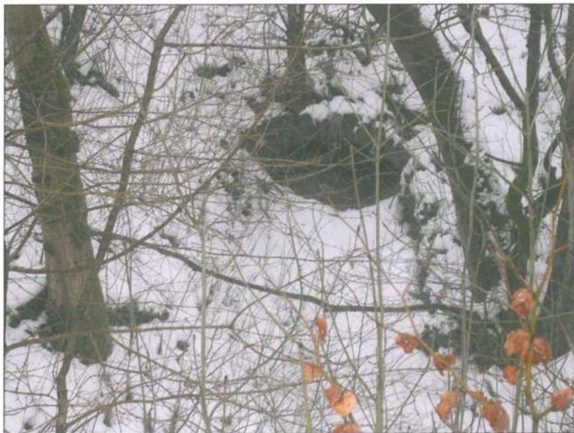
Plate 91. Arched level or culvert entrance EA099.05, view to east
