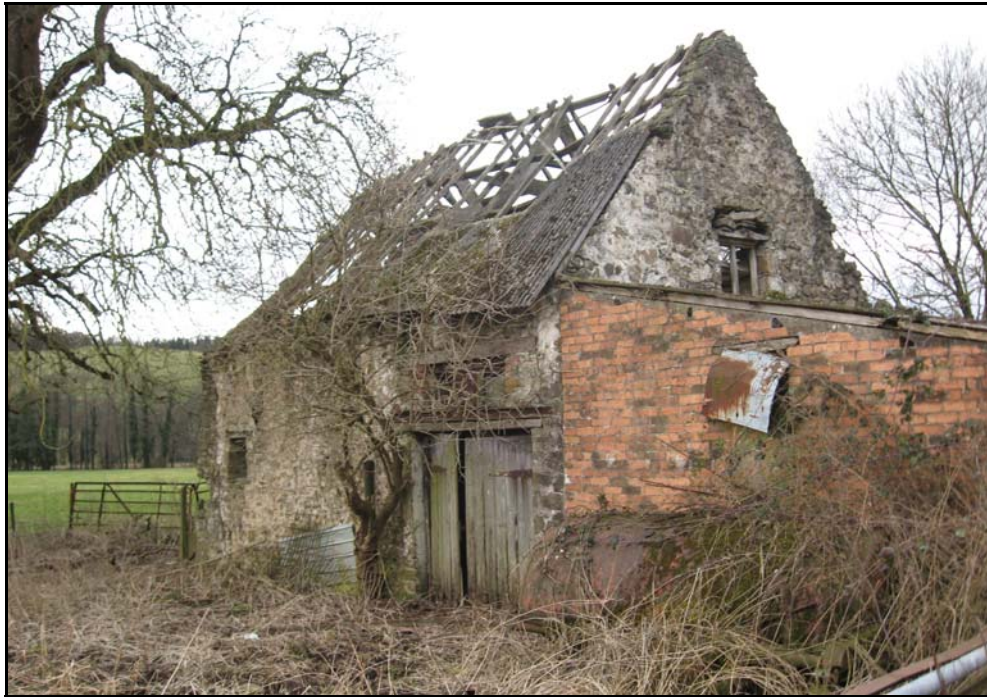
Plate 109: SW elevation of Machen Mill (MP027). View to W.
