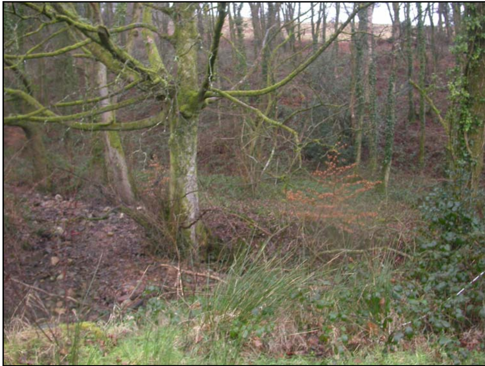
Plate 102: General view of recorded location (NGR SS 57028 95669) for Cwm Rian, Cefn Golau Mill (MP012). View to SW.
