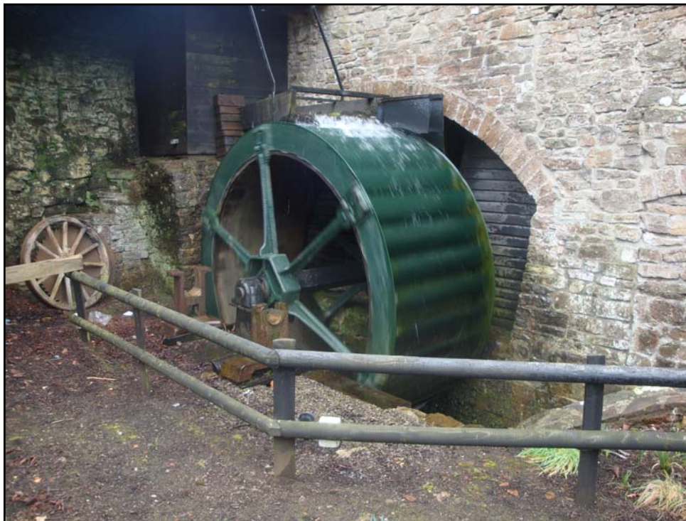
Plate 86: View of the wheel SE elevation at the Water Wheel (PRN 05687g). View to W.
