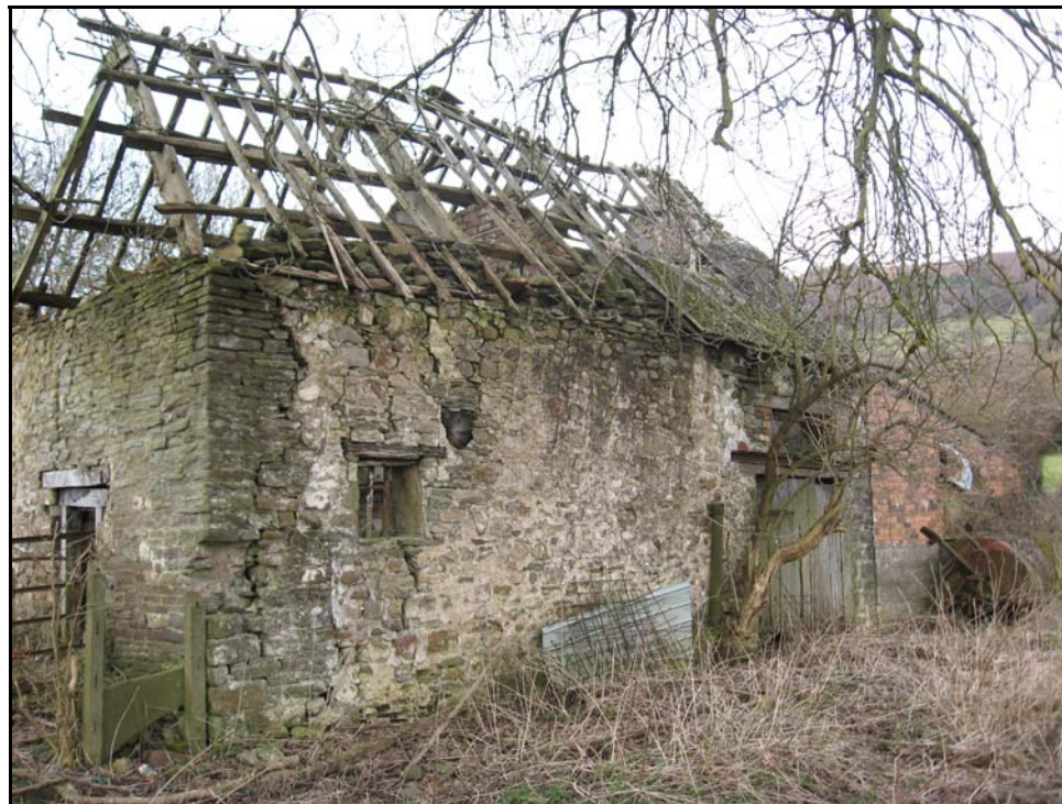
Plate 108: SE elevation of Machen Mill (MP027). View to NW.
