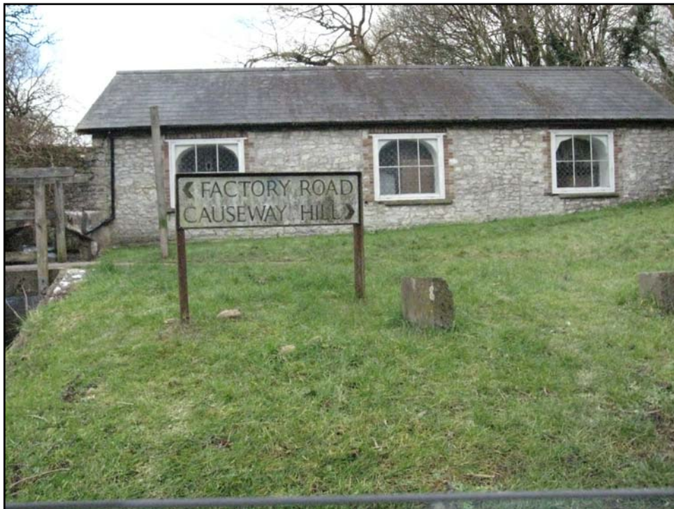
Plate 37: View of factory close to mill near Cowbridge with Llanblethian (PRN 04012s). View to W.
