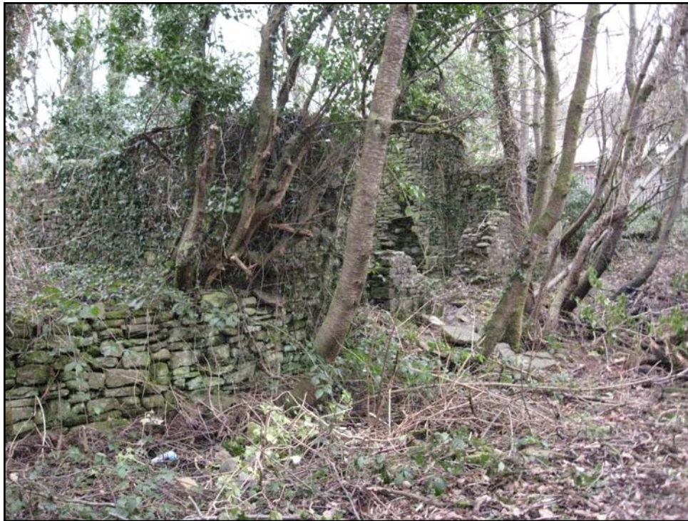
Plate 15: View of external SE elevation of Old Mill Ystrad (PRN 00929m). View to N.
