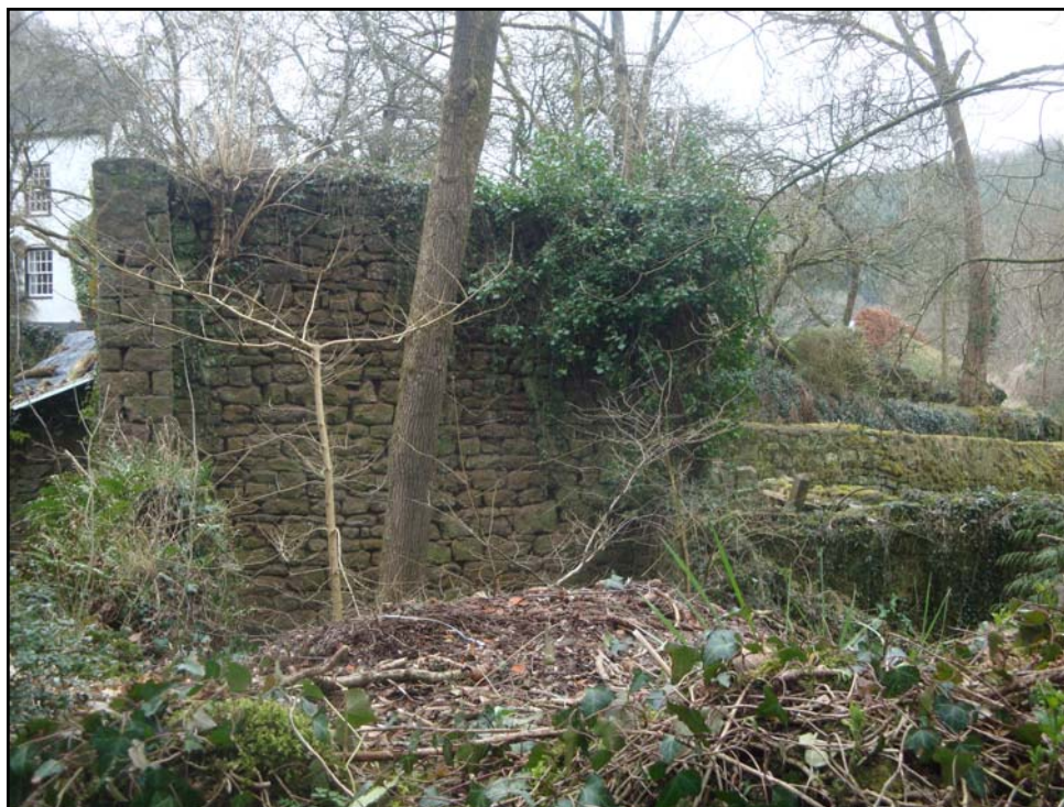
Plate 95: View of possible mill structure of The Glynn Paper Mill (PRN 07967g). View to N.
