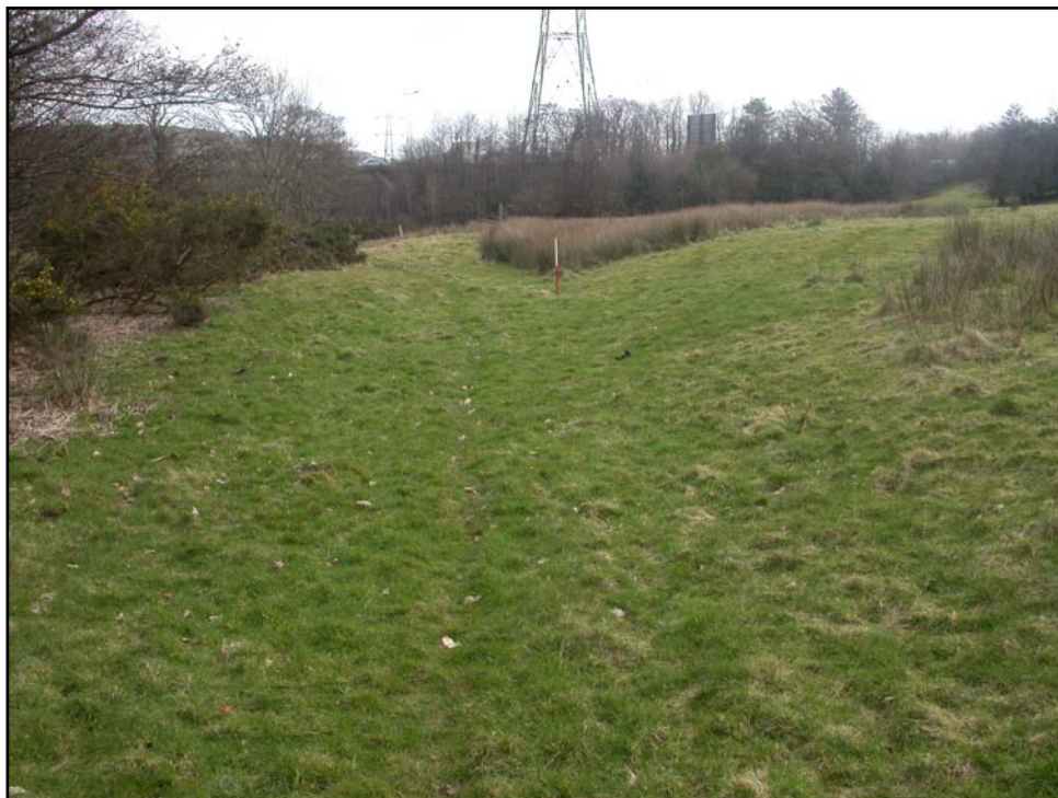
Plate 32: View of leat (01079.0m) running northeast southwest at Afon Clun Mill (PRN 02217m). View to NE.
