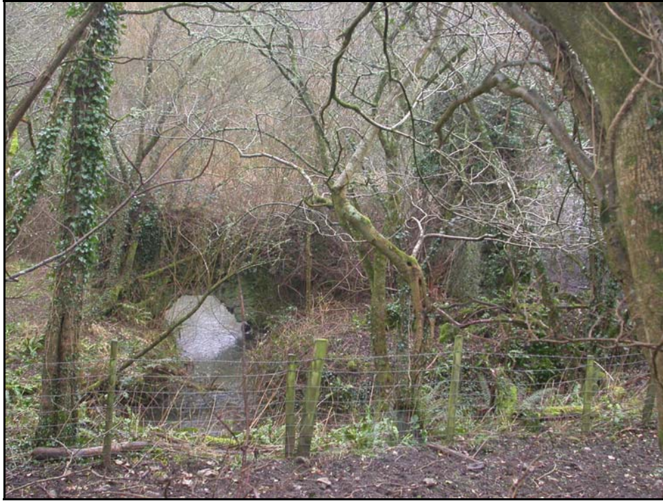
Plate 100: General view of Leason Mill (MP008). View to N.
