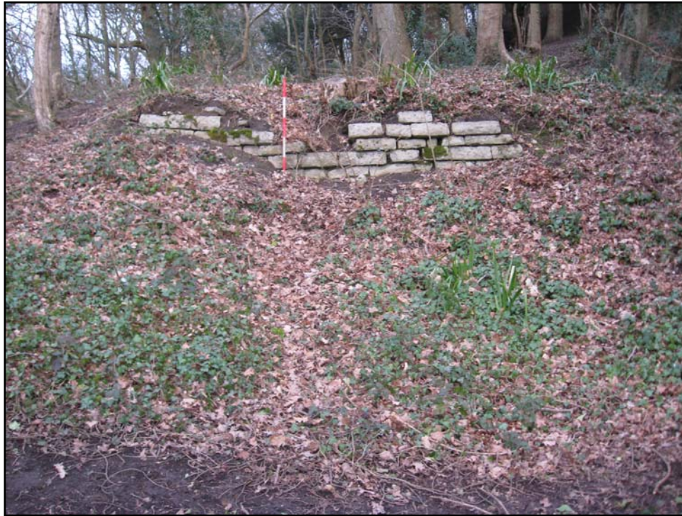
Plate 7: View of the stonewall and depression at Porthkerry Park Mill (PRN 00695s). View to NE.
