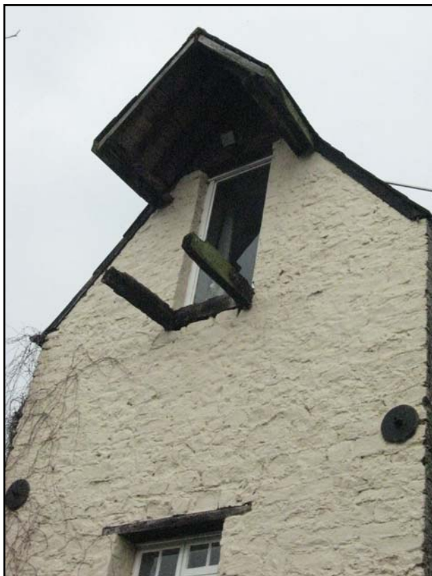
Plate 28: Detail of the flour shoot at Llanfythyn Mill (PRN 01993s). View to NW.
