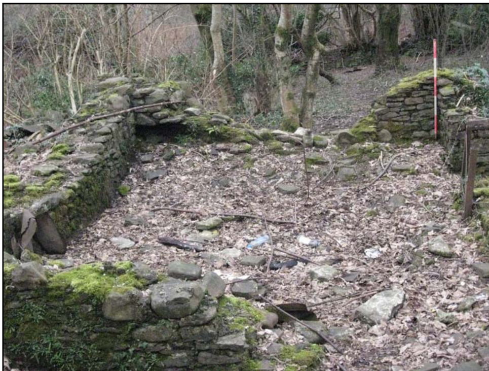
Plate 20: View of the rooms at Old Mill Ystrad (PRN 00929m). View to NW.
