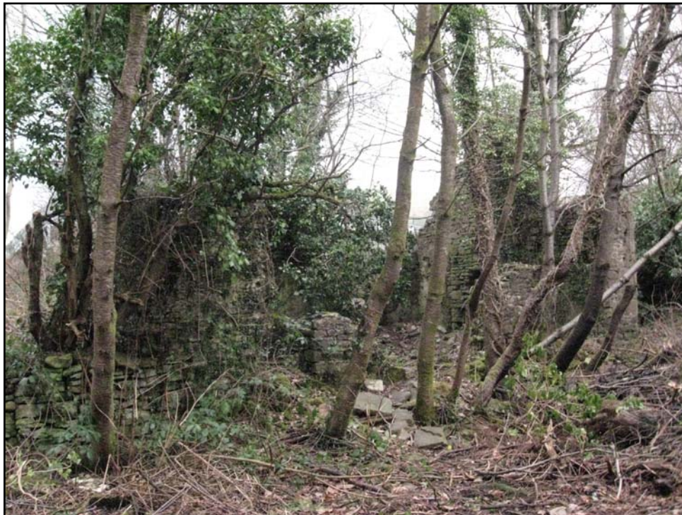
Plate 16: View of external SE elevation of Old Mill Ystrad (PRN 00929m). View to NW.
