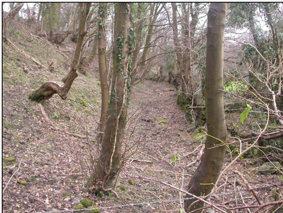
Plate 47: View of mill race from the road at Llanmihangel Mill (PRN 02876w). View to E.
