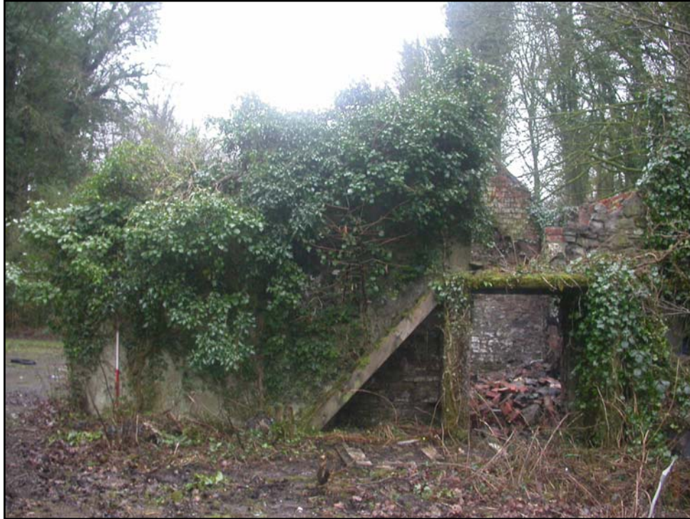
Plate 25: View of the southwestern group of structures at Neath Abbey Mill (PRN 01869w). View to SW.
