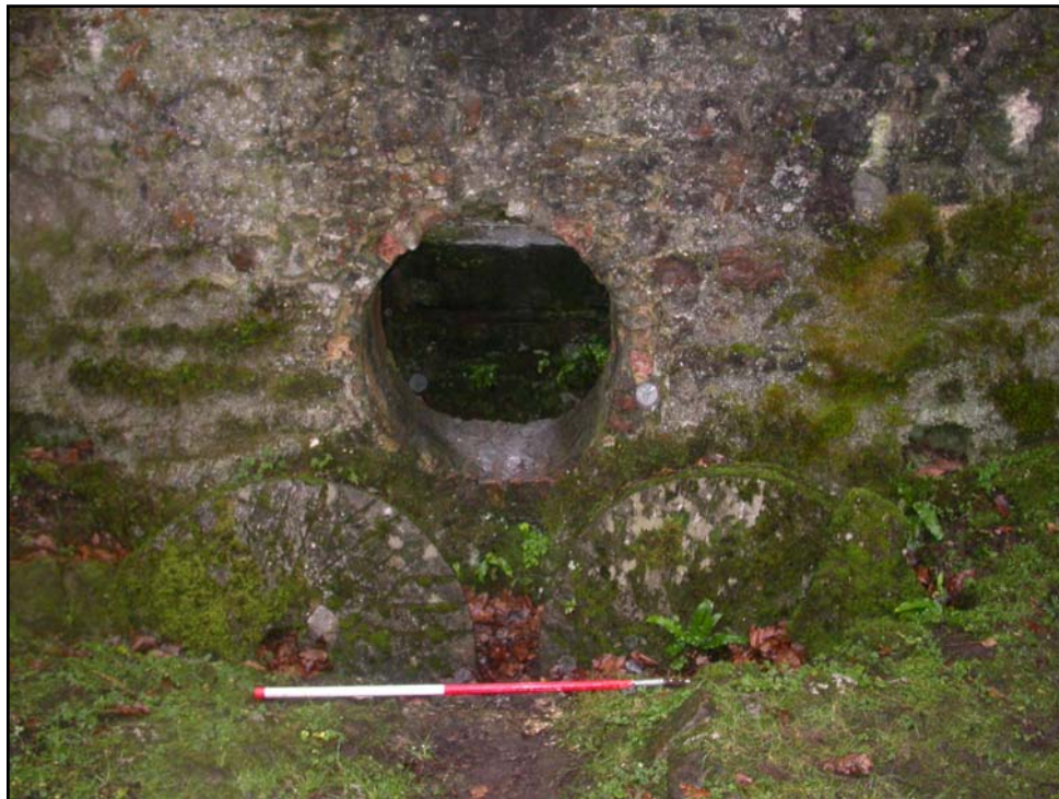
Plate 59: View of the millstones and wheel beam pole at Penrice Mill (PRN 03818w/00823w). View to W.
