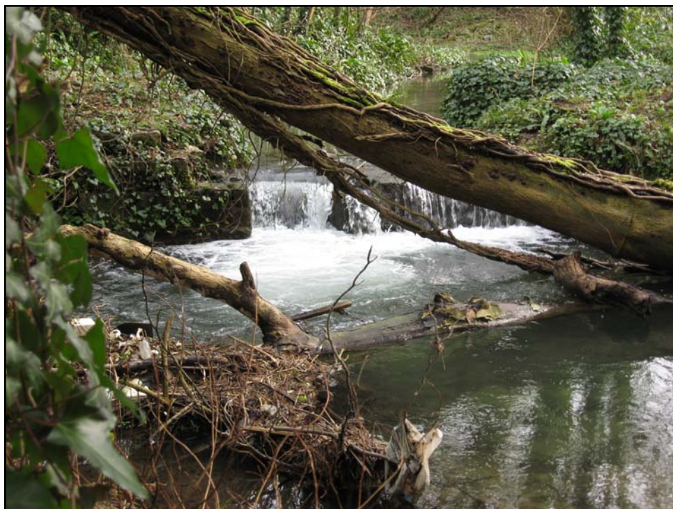
Plate 33: View of weir at Corn Mill (PRN 02369s). View to E.
