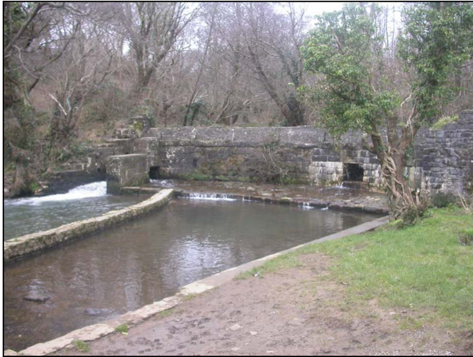
Plate 45: View of dam at Llanmihangel Mill (PRN 02876w). View to NE.
