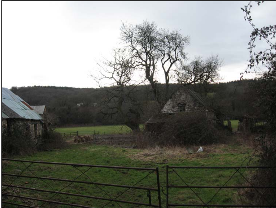
Plate 107: General view of Machen Mill (MP027). View to SW.
