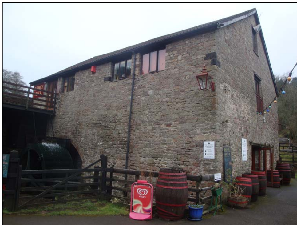
Plate 84: View of the SE facing elevation at the Water Wheel (PRN 05687g). View to W.
