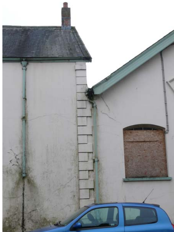
Photograph 13 Building A, Ashlar Facing on West Gable Corner
