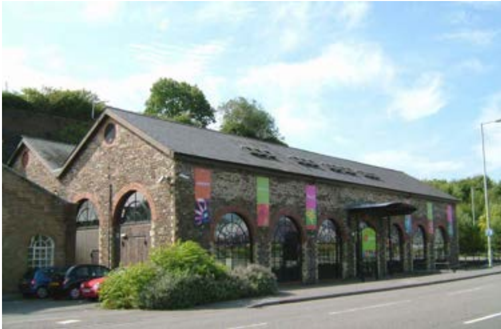
Plate 014: Former stores building or casting shed, Gadlys Ironworks (Listed Grade II), view to northwest.
