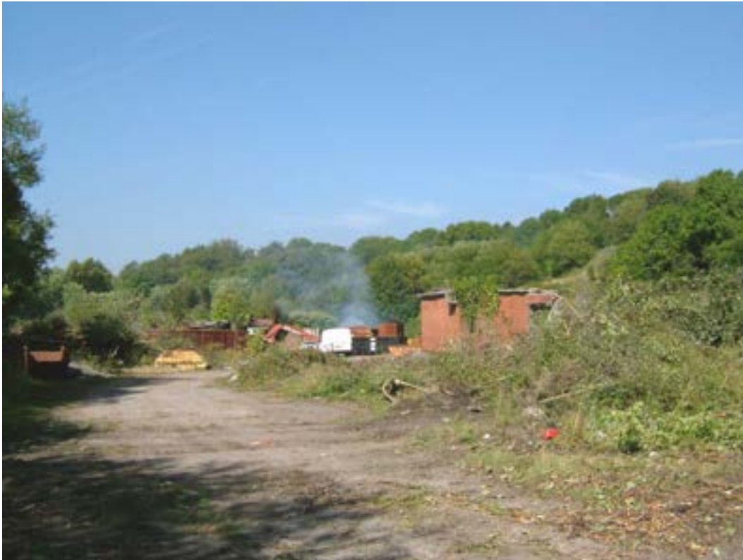
Plate 013: Llwydcoed Ironworks site with clearance activity in progress, view to northwest. Furnace site lies within wooded area beyond redbrick structure on right hand side of the picture.
