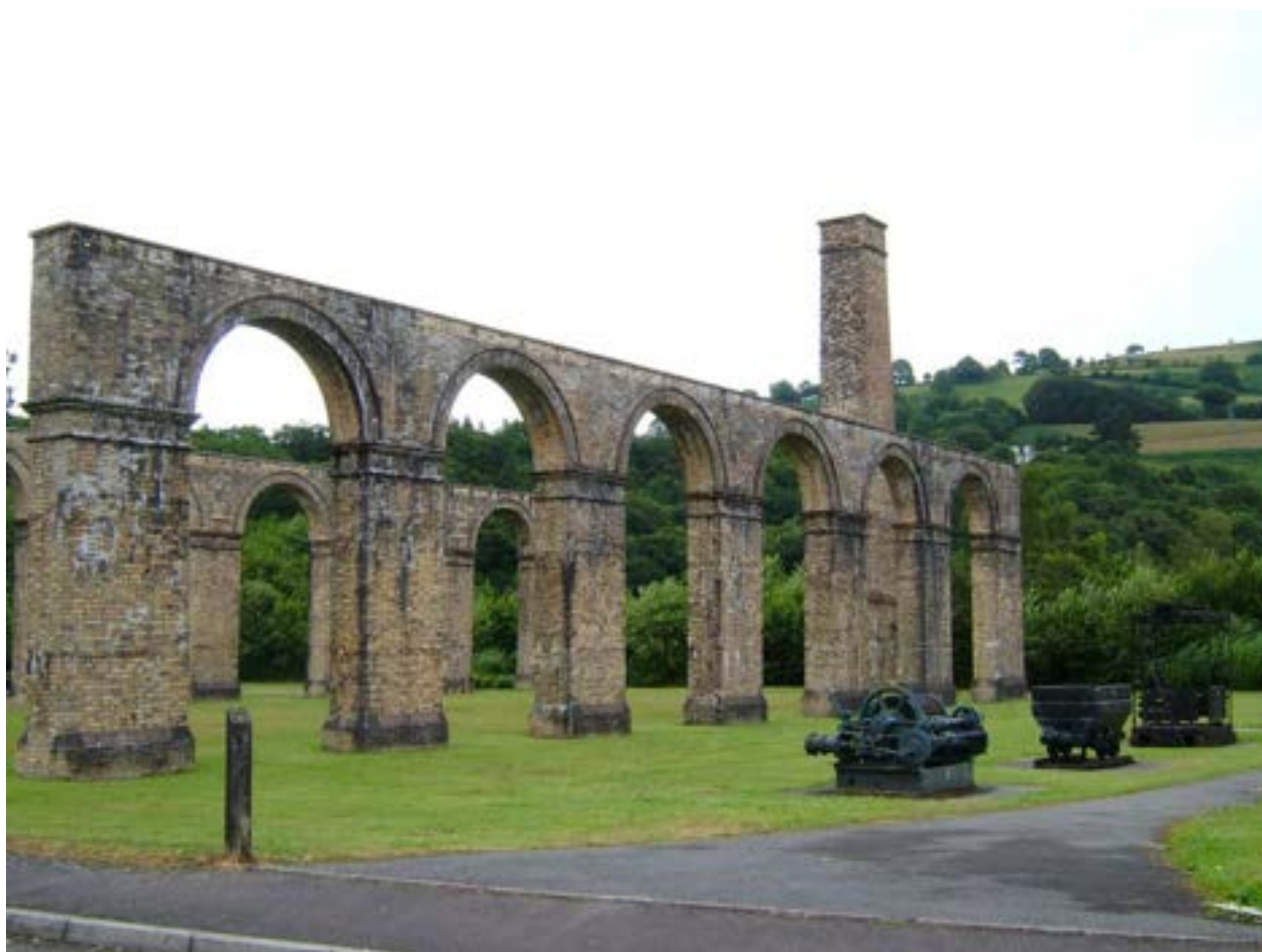
Plate 018: Remains of the mill/engine house (NPRN 34,037) at Ynyscedwyn, view to southeast.
