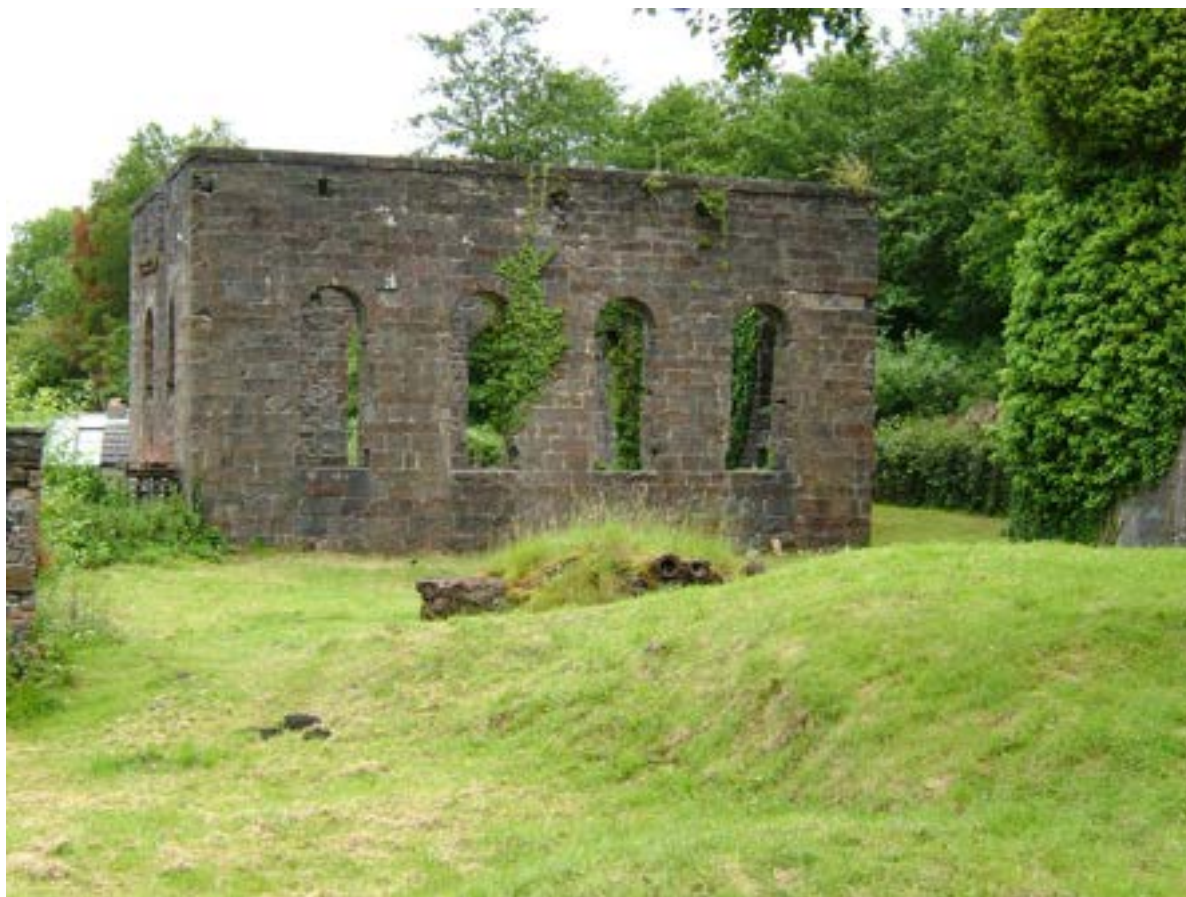
Plate 022: Remains of the Engine House (PRN 04295w), Venallt Ironworks (SAM Gm423), view to northeast.
