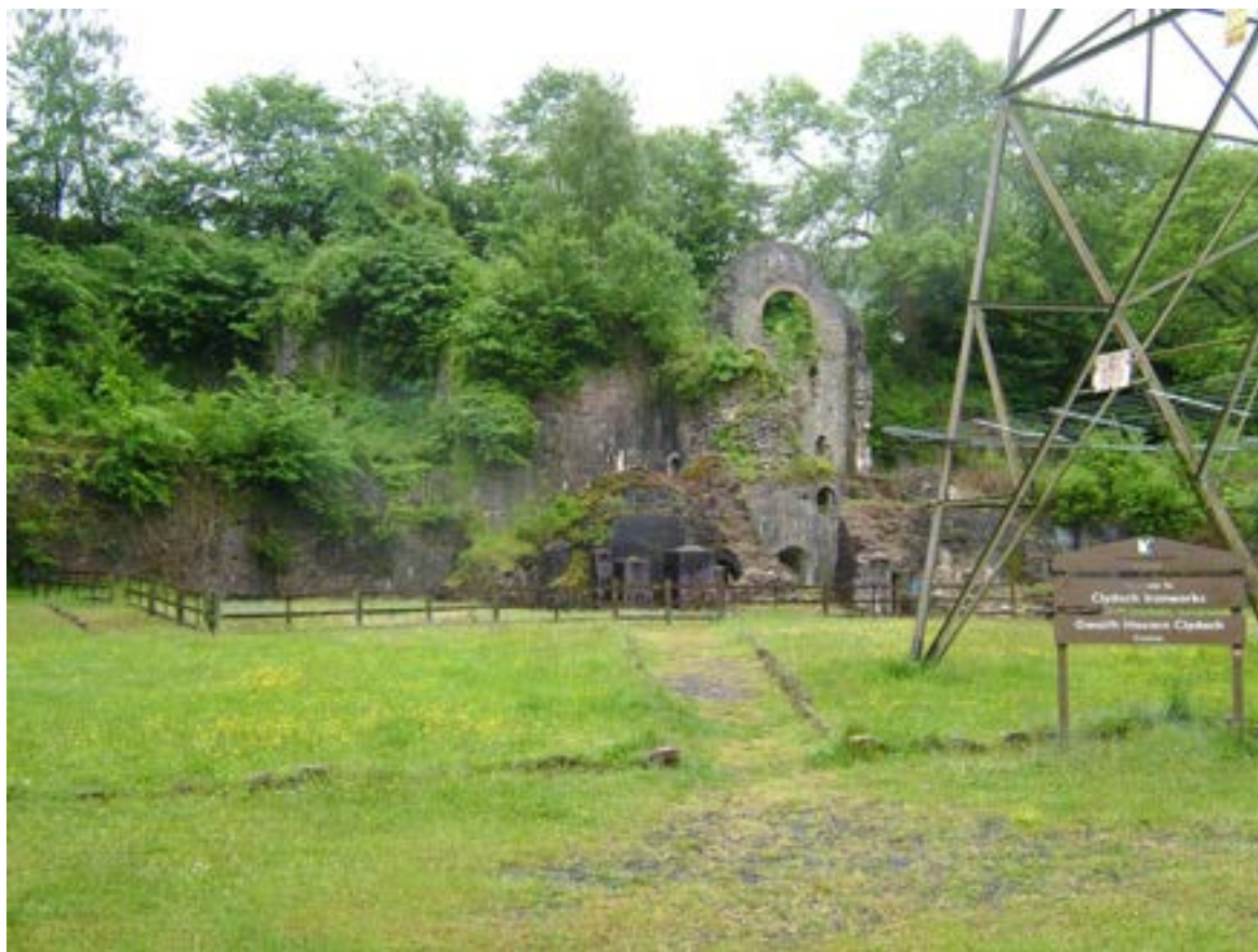
Plate 003: General view of the Clydach Ironworks (PRNs: 02476g and 03647g; NPRNs: 34,030 and 306,268; SAM BR161), view to the southwest.
