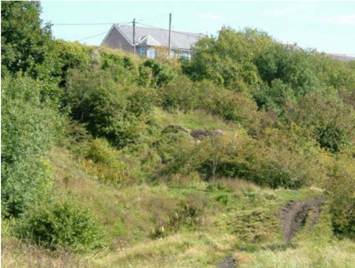
Plate 012: Furnace bank site Hirwaun Ironworks (SAM BR157), view to northeast. The entire area including the scheduled remains is in an increasingly derelict and overgrown state.
