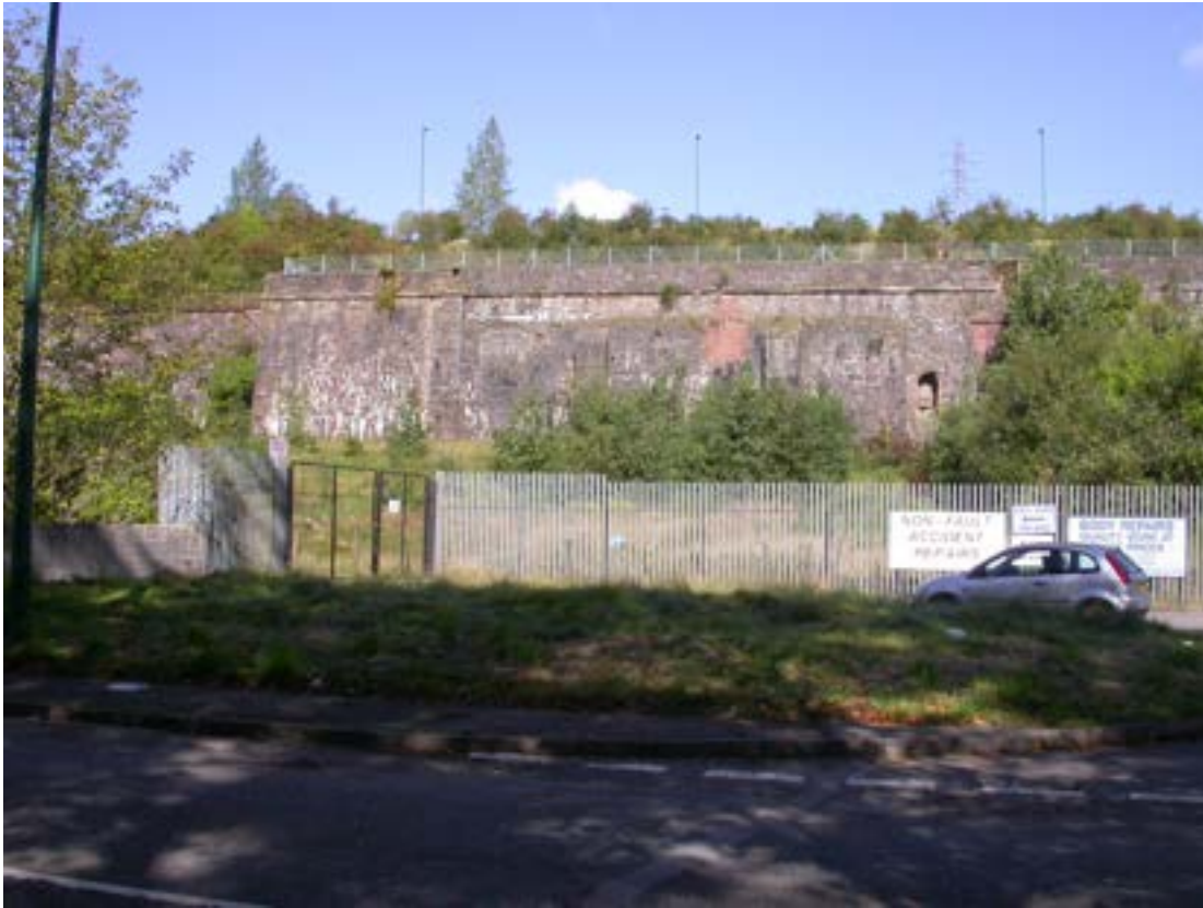
Plate 006: The Grade II* listed furnace bank site (Cadw ref: 22531) at Ebbw Vale Ironworks (IW010a) view to east.
