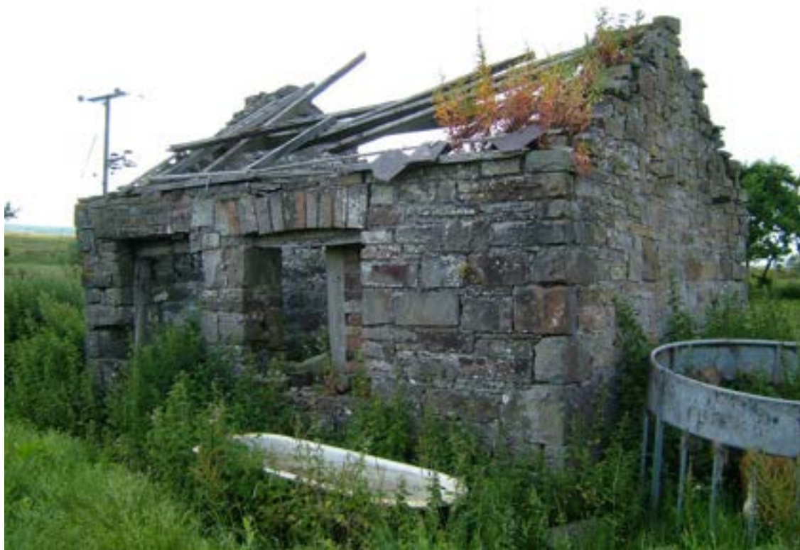
Plate 020: Remains of the Weighbridge House, Banwen Ironworks, view to northwest.
