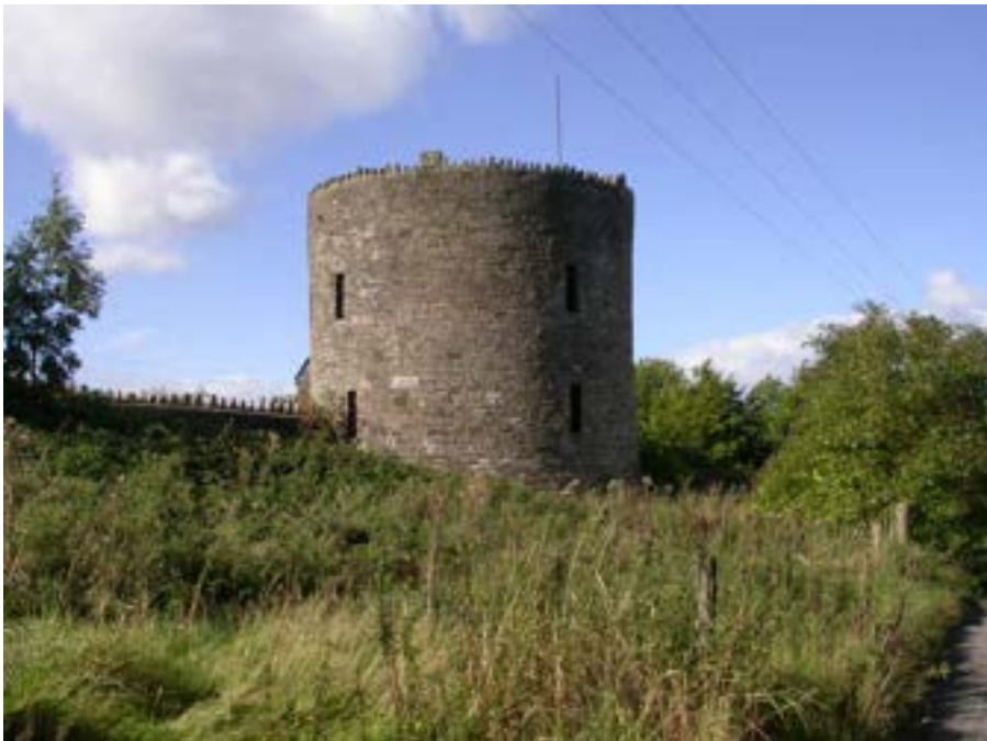
Plate 005: View towards the NE Roundhouse, Nant-y-glo Ironworks (IW009b) view to northwest.
