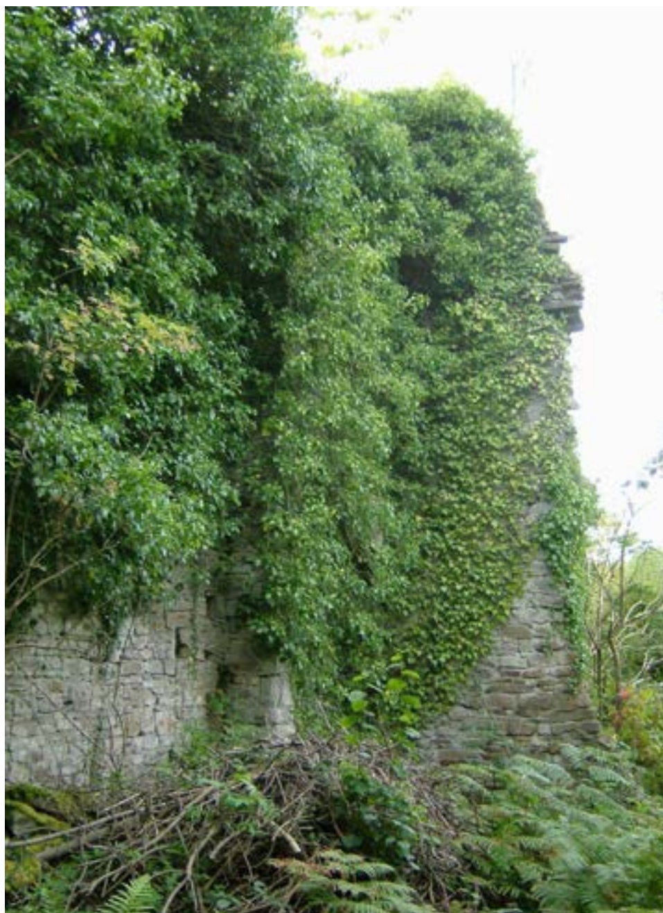
Plate 021: Standing remains Melincwrt Ironworks (SAM Gm416), illustrating overgrown nature of the site, view to north.
