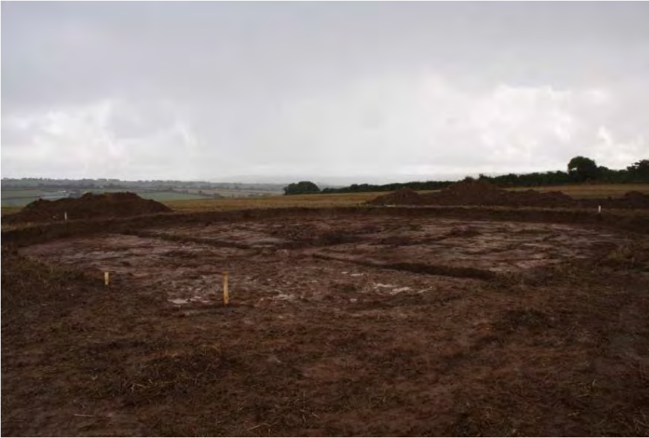
Photo 1. Excavation area opened across Bronze Age barrow PRN 55928 after machining has been completed, looking southeast.
