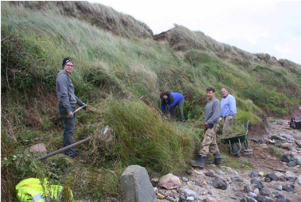
Photo 1: Initial clearance of the sand dunes
